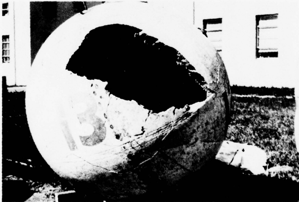
Figure 18. This view of Sphere no. 13 is typical of post-implosion for non-preloaded spheres. The missing concrete was pushed to the interior of the sphere. Shear-compression plane runs from equator to above the numeral 13.
