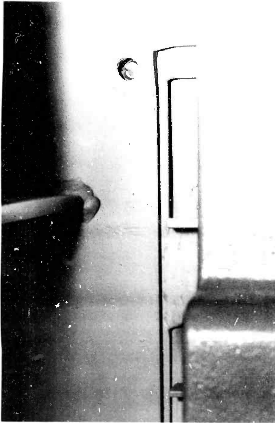
Fig. 57 - Damage from Shock Test - 1600 A Breaker Bay (Rear). Sheared bolt supports upper end of the lower 1600 A Breaker base.
