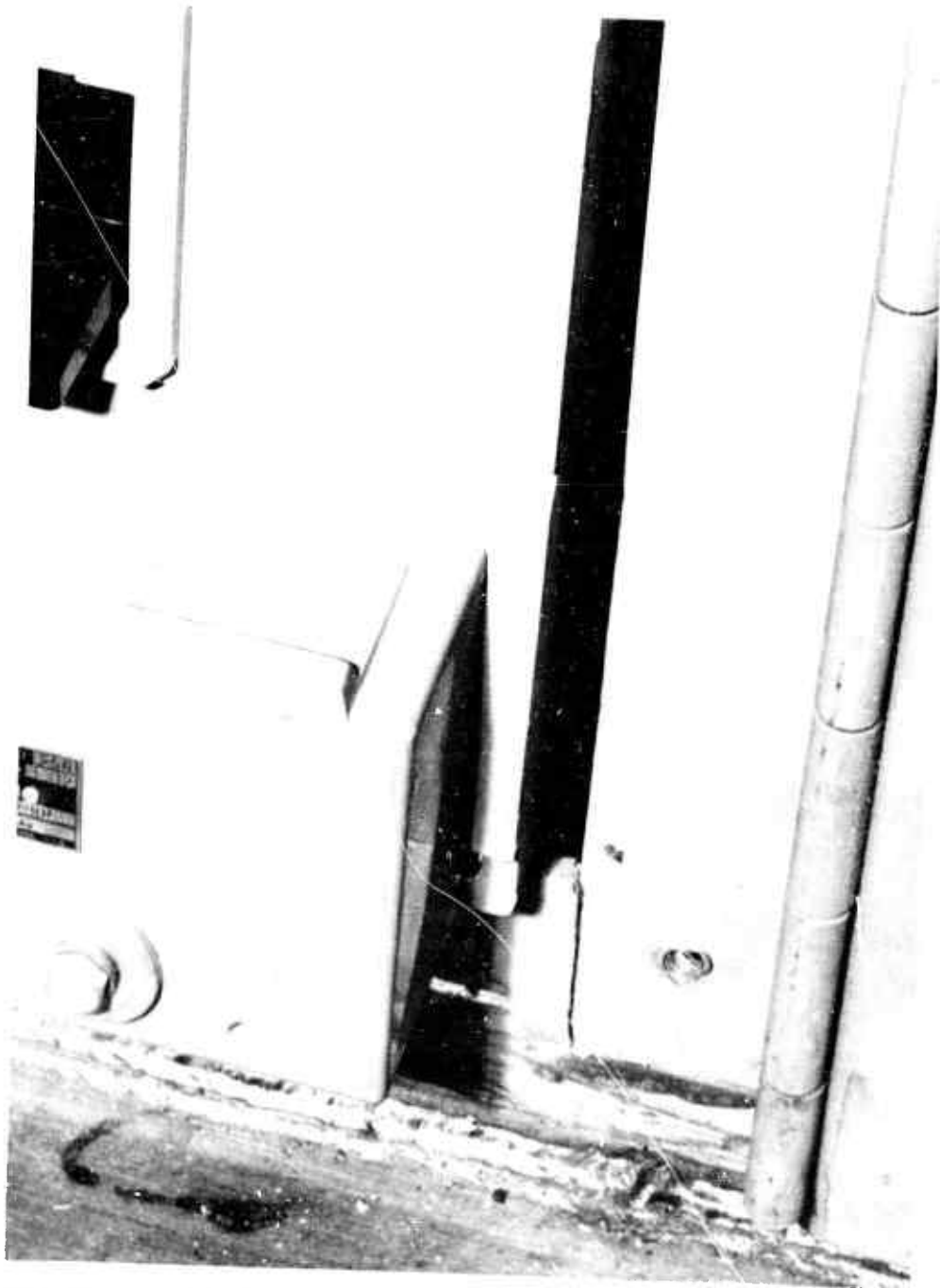
Fig. 49 - Damage from Shock Test - AQB Breaker Bay. Inner vertical frame member broken loose at base, and horizontal bottom member shifted over.
