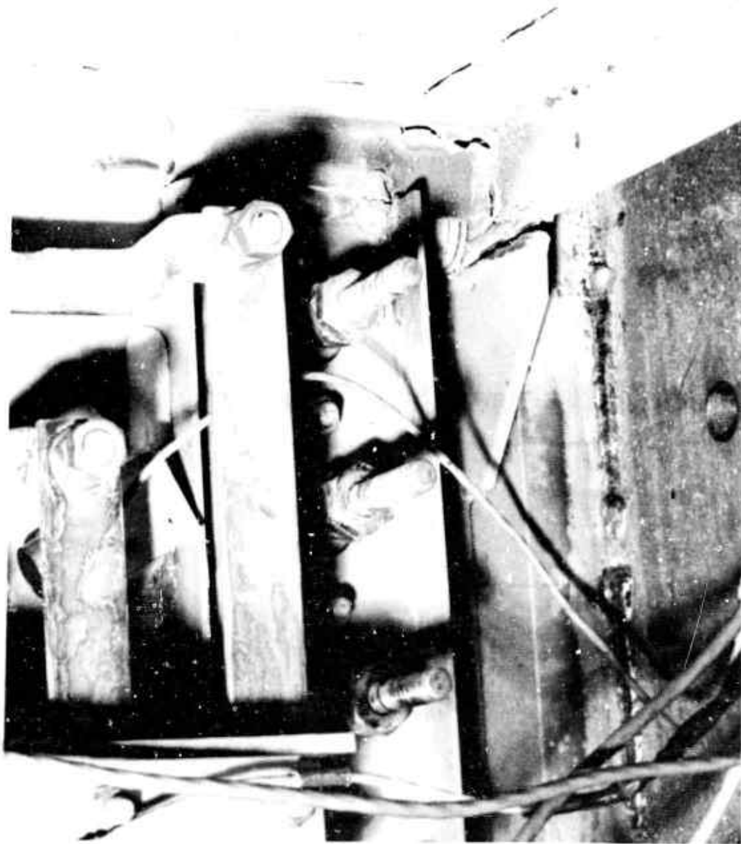
Fig. 64 - Damage from Shock Test - AQB Breaker Bay (Rear). Broken welds in frame base structure, outboard end.
