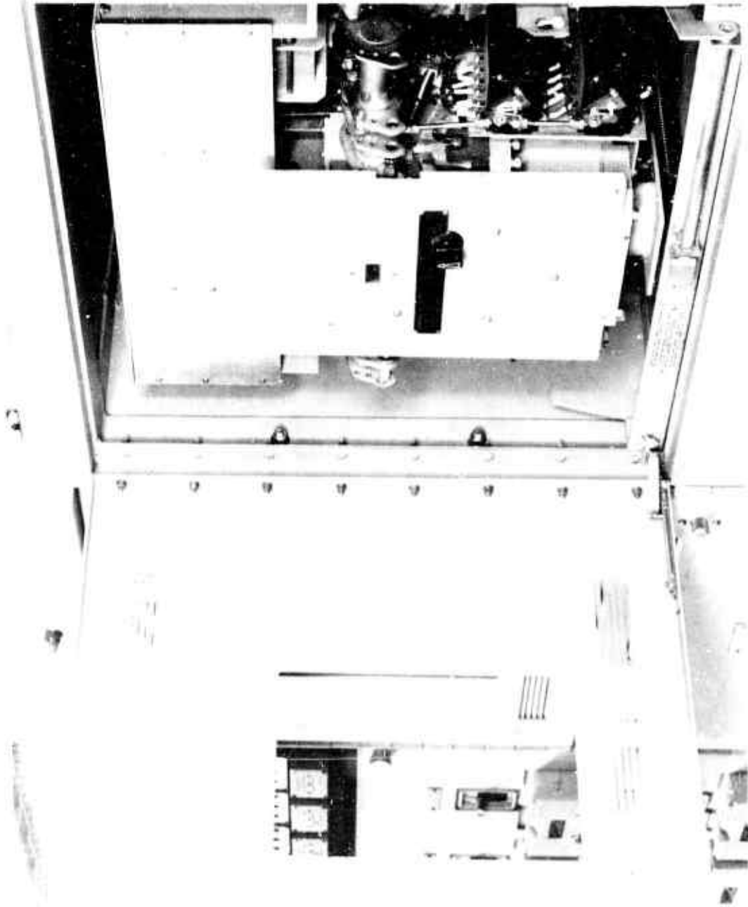
Fig. 18 - Damage from vibration test - ACB-2400. Note abrasion of breaker and door, and bending of louvers.
