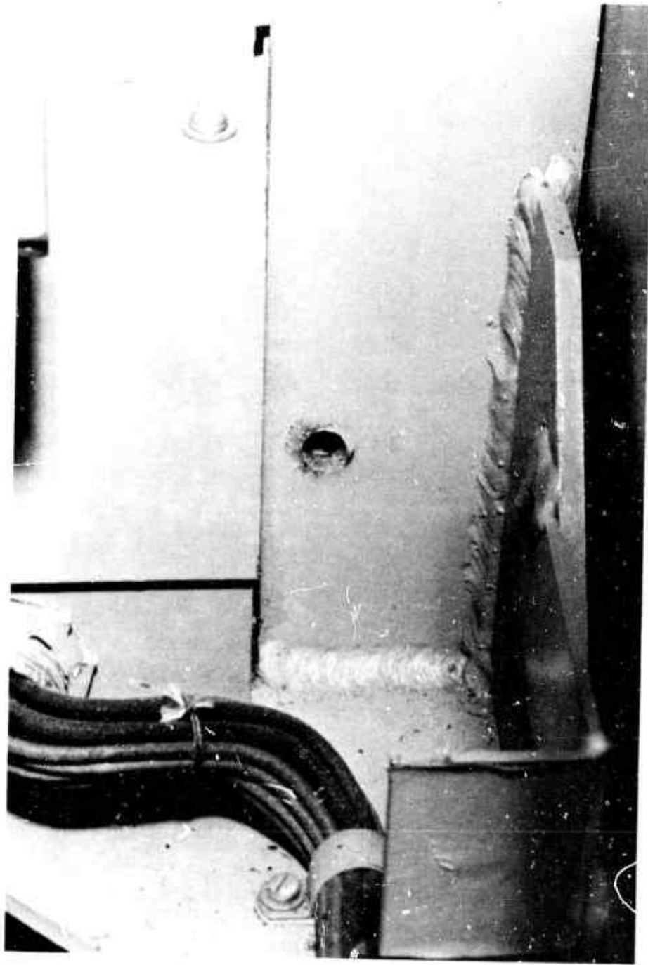
Fig. 58 - Damage from Shock Test - 1600 A Breaker Bay (Rear). Sheared bolt supports lower base frame for the lower 1600 A Breaker.
