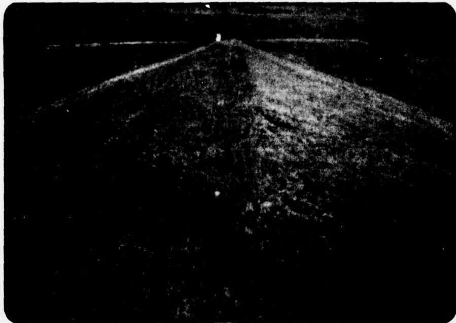
Photograph No. 1 Crest (looking west).
