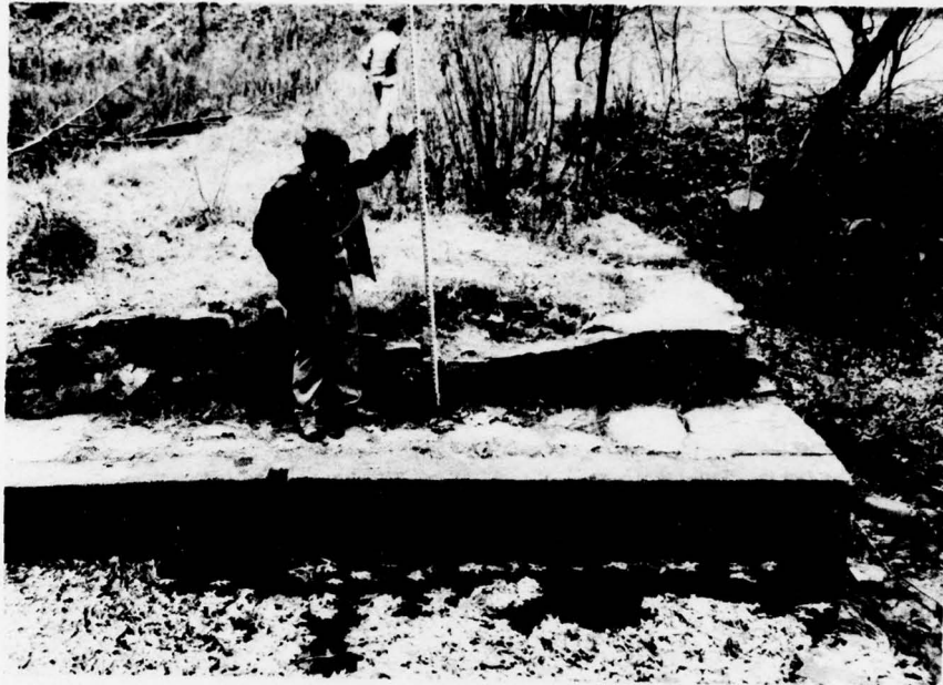
E. Spillway Left Wall.
