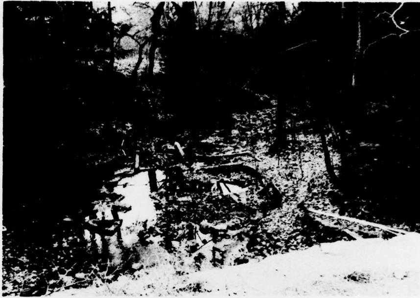
I. Channel Downstream of Dam.
