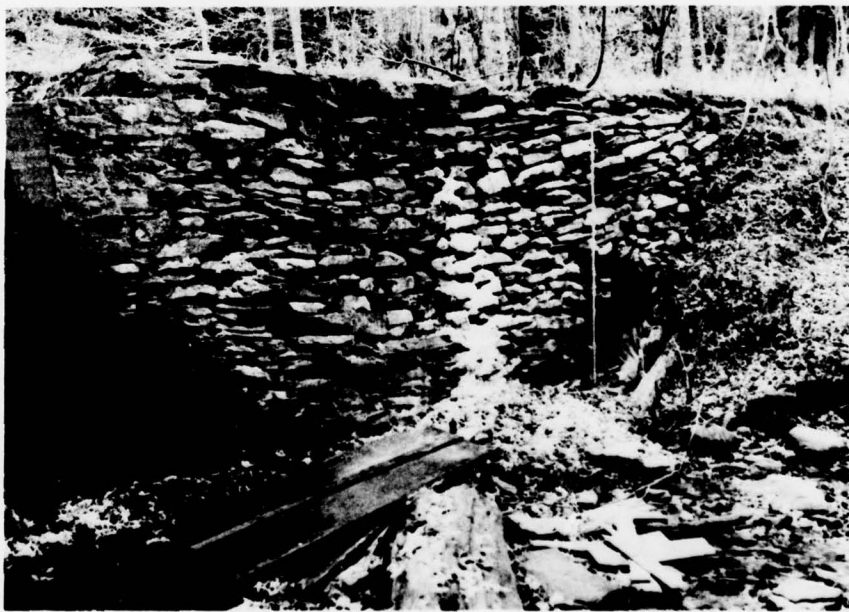
H. Downstream Face of Dam to Left of Spillway.
