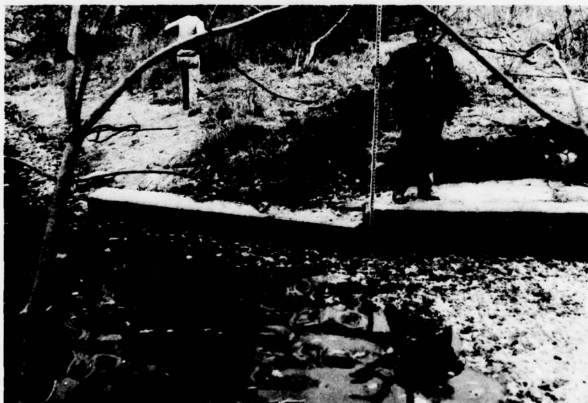
D. Spillway Left Approach Wall.
