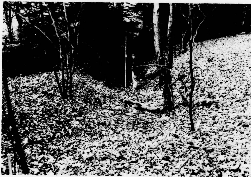
F. Auxiliary Spillway Channel.
