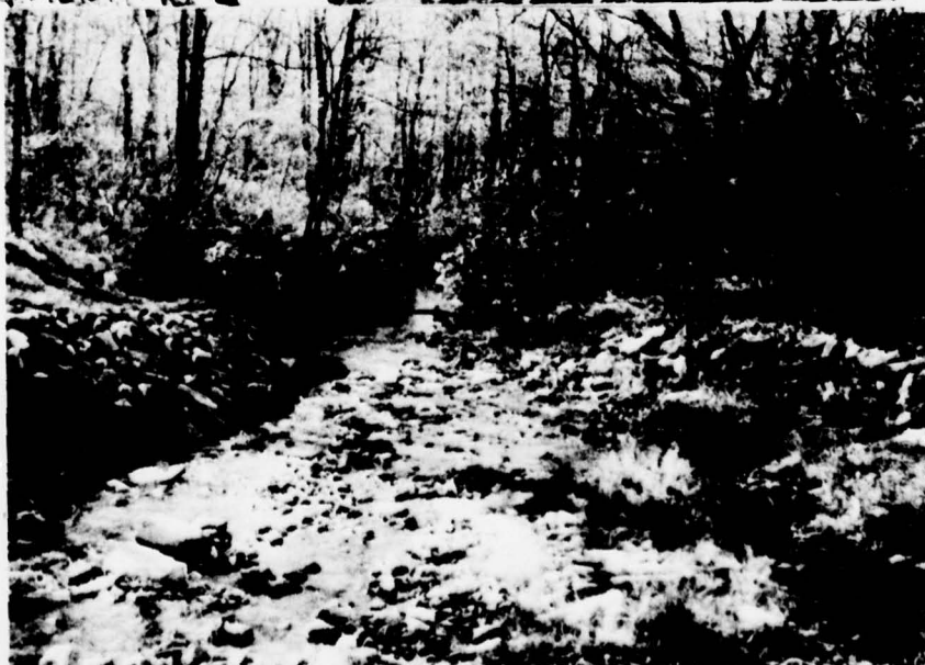
Spillway Outlet Channel
