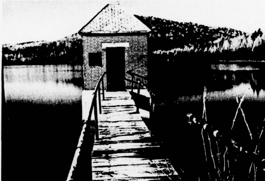
PHOTO 9. View of Intake Tower and Walkway
