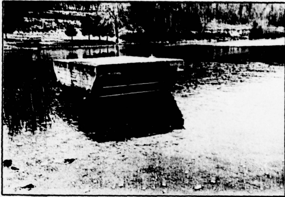
PHOTO 3. Close-up of Intake Riser
