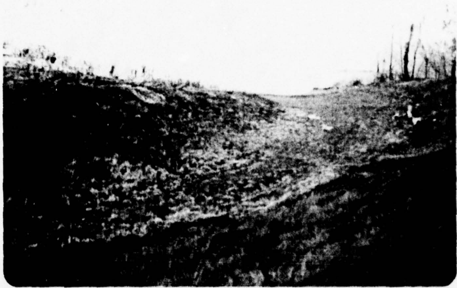
Photograph No. 1 Emergency spillway approach channel.
