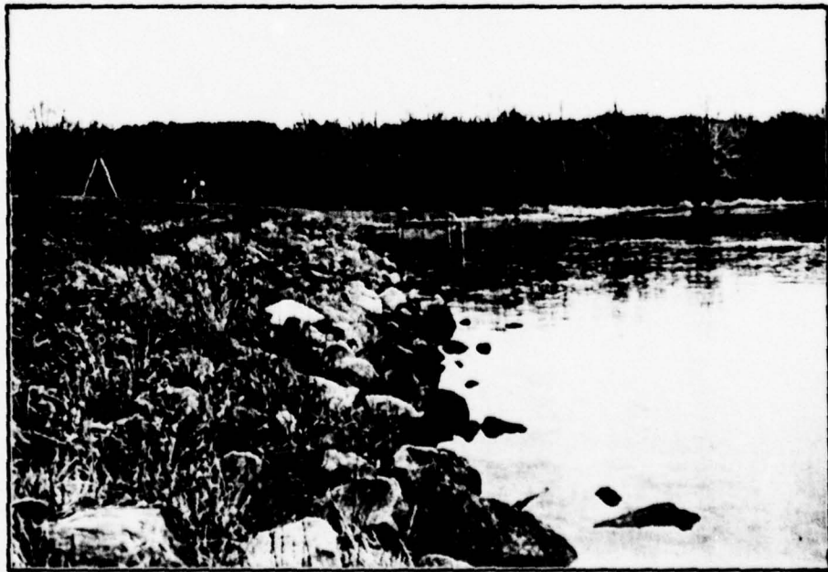
PHOTO 2. View of Principal Spillway Intake, Upstream Slope, and Riprap Protection
