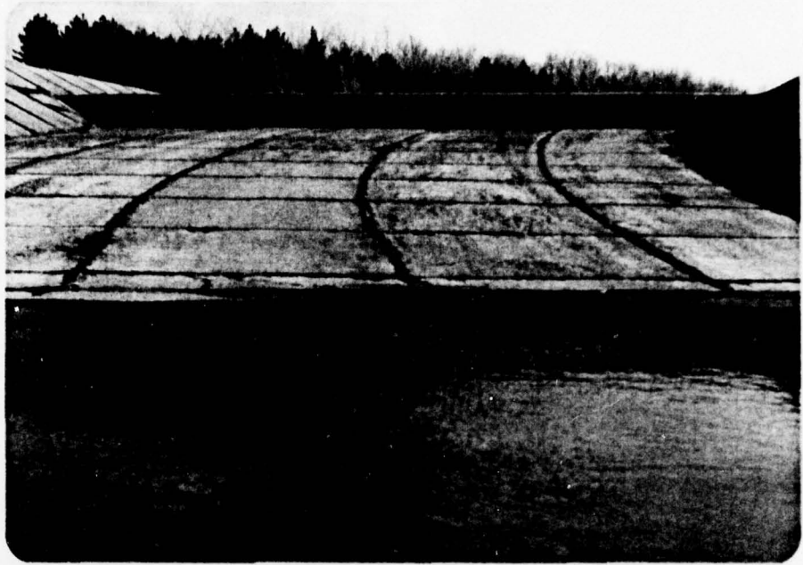
Photograph No. 3 Spillway discharge channel.
