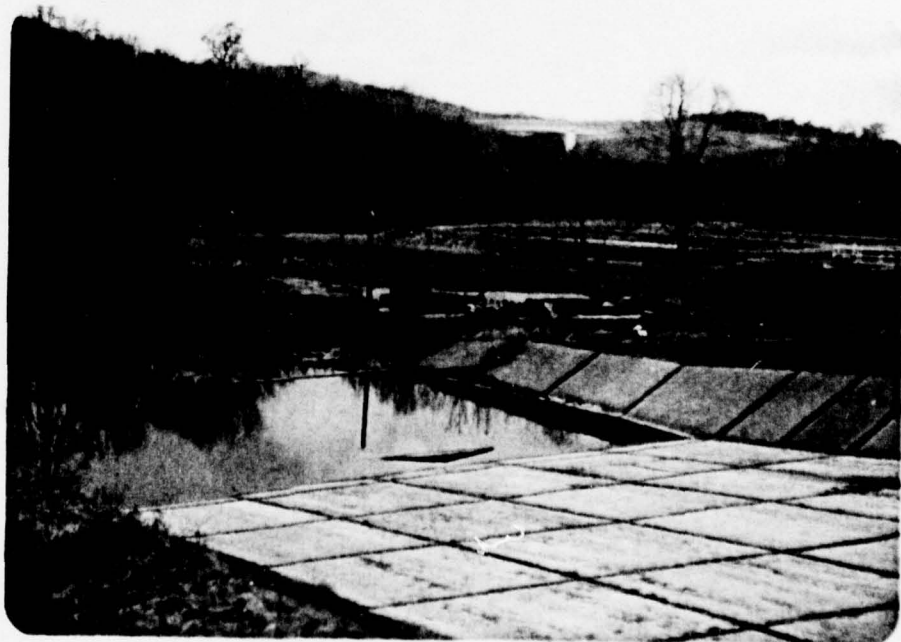
Photograph No. 4 Spillway stilling basin.
