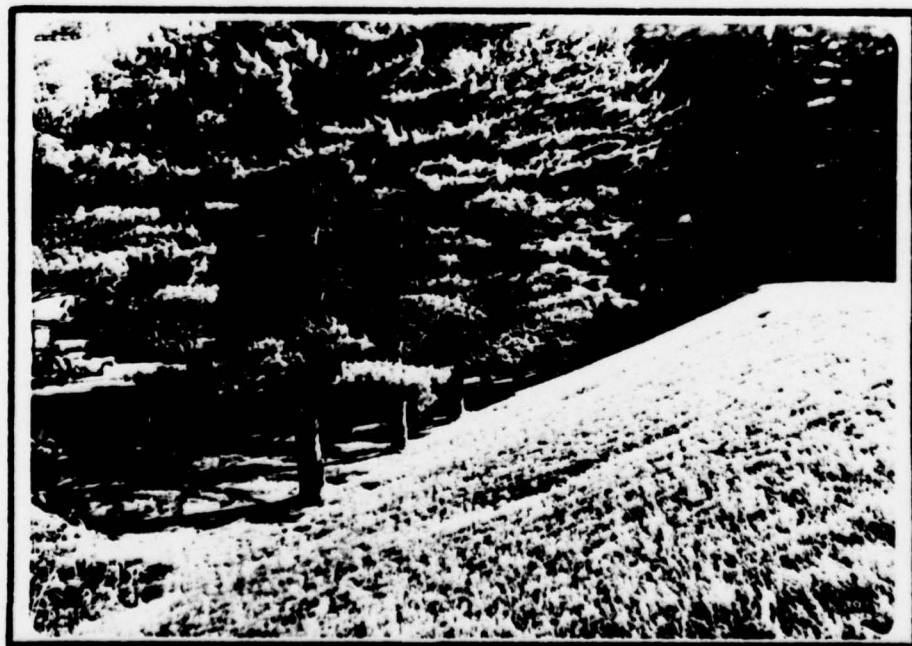
Downstream slope from left abutment.
