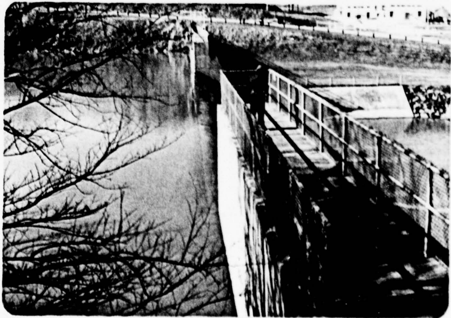
Photograph No. 2 Crest (looking west).
