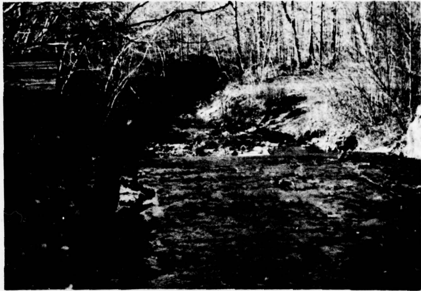
Spillway Outlet Channel
