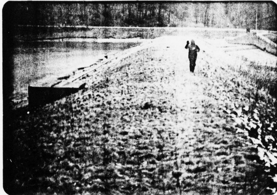
Photograph No. 1 Crest (looking north).
