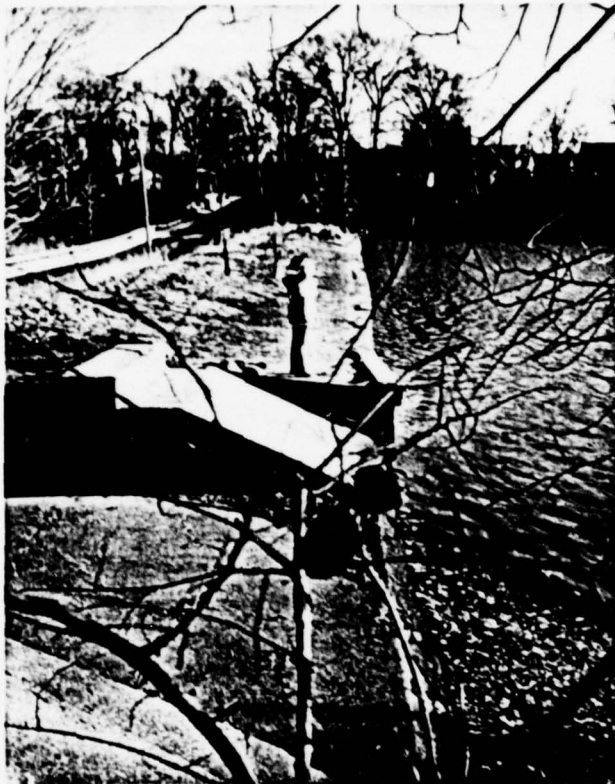
Auxiliary Spillway (Looking South)
