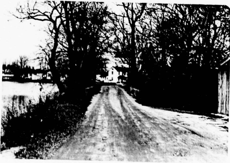
PHOTO 10 Hearns Pond Mill Road Over Embankment and Dams - 7140 Feet Upstream of Williams Pond
