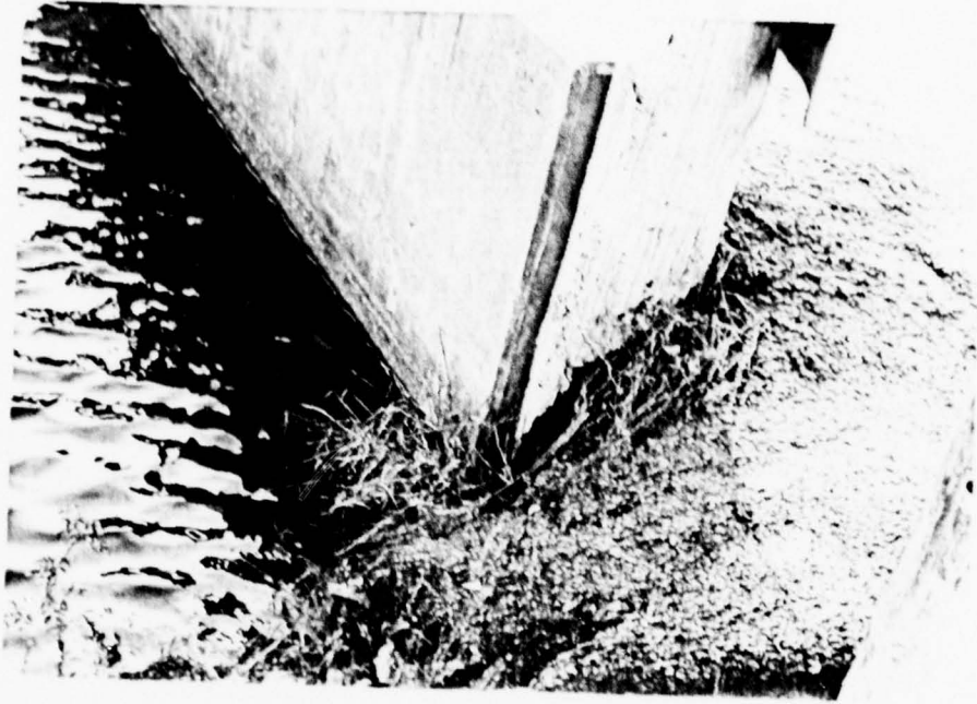
PHOTO 9 Bituminous Paving Installed To Correct/Prevent Erosion-Williams Pond
