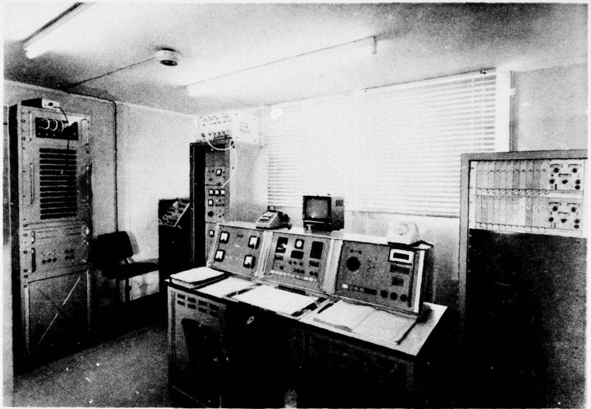
FIG 5 CONTROL ROOM FOR 40 FT EARTH STATION
