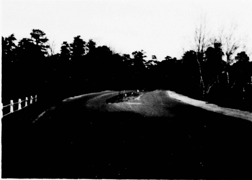
PHOTO 9 ROADWAY ON CREST OF DAM
