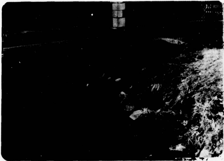
Deteriorated riprap at right. 7 December 1978 abutment.
