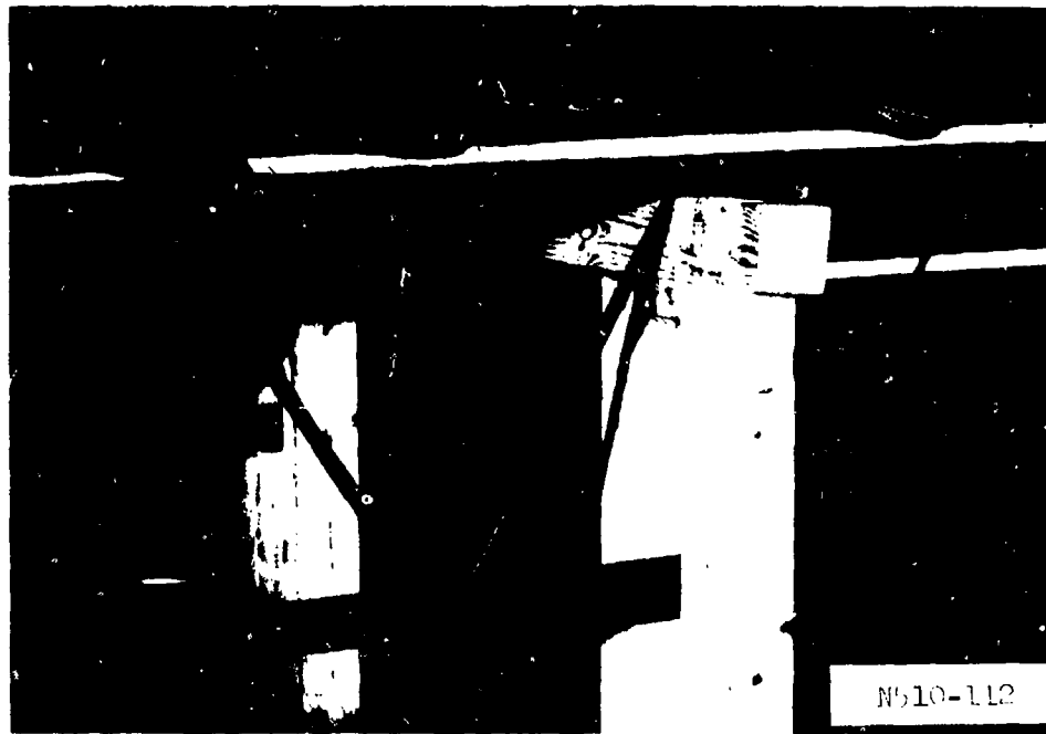
B. Closeup of Connection Between O.W.J. and Supports.
