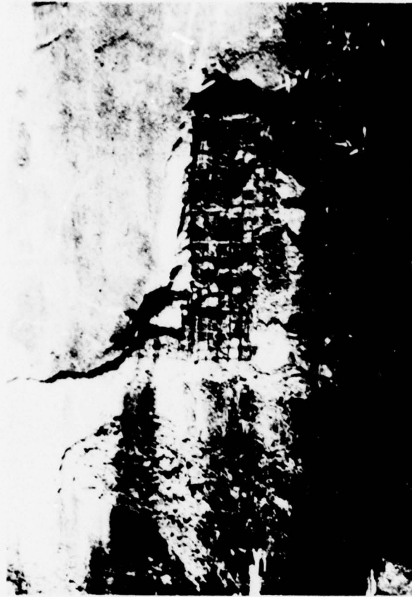
FIGURE 15 DETAILS OF SPALL ON LEFT ABUTMENT DOWNSTREAM WINGWALL
