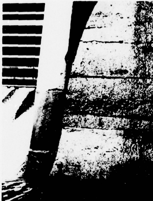
FIGURE 5 CRACKS IN LEFT GRAVITY/SPILLWAY SECTION NEAR PIER 4
