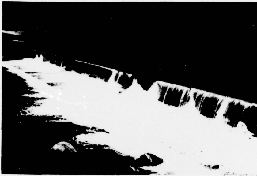
FIGURE 19 TEMPORARY IMPOUNDMENT DAM AT STATE CAMPSITE
