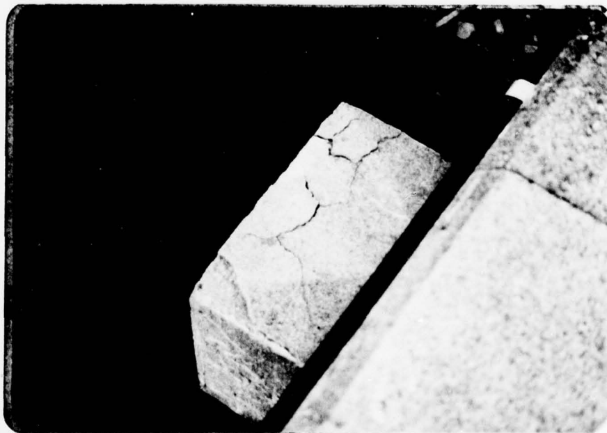
Pier supporting footbridge. Note: deteriorated concrete.
