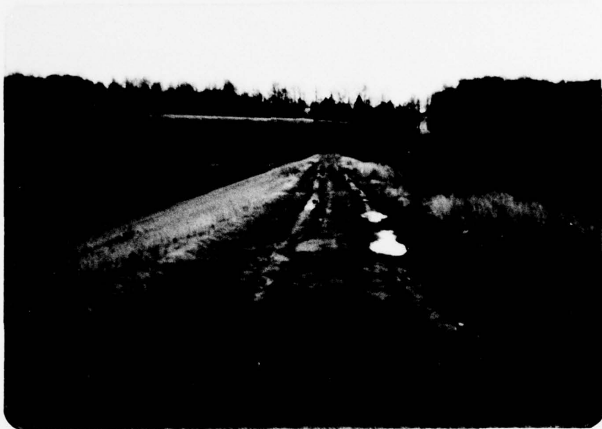
Crest of earthfill dam. Note sags in crest.
