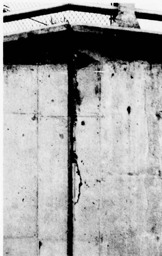
RETAINING WALL JOINT WITH SPALLING ALONG STORM WATER FLUME
