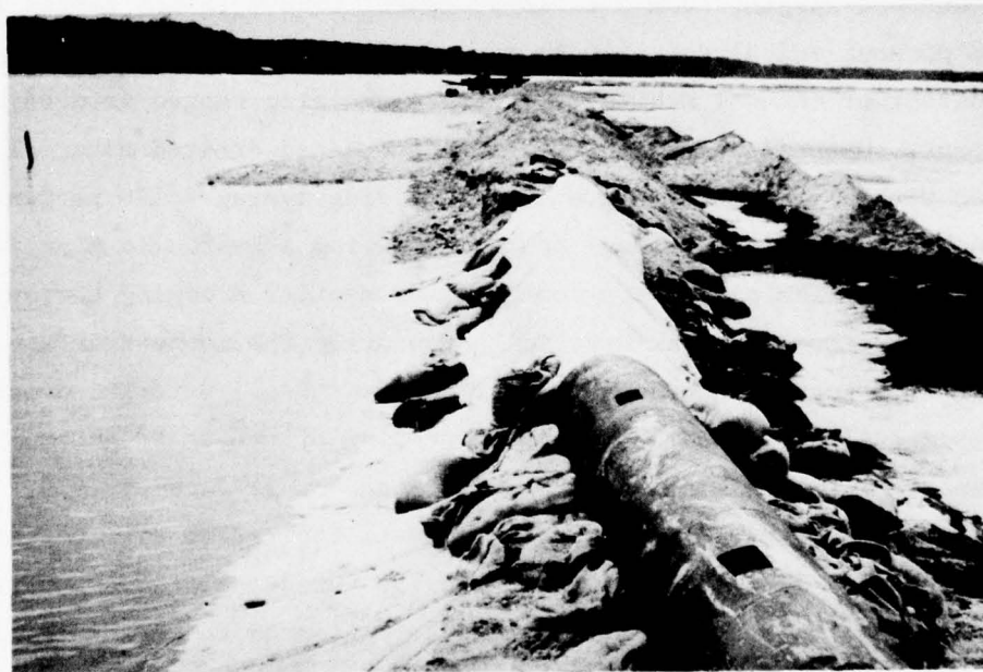
b. REPAIRED BREACH, 29 JAN 1975
