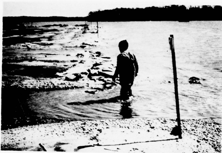
Figure 13. Breached section along south dike, 25 Mar 1975
