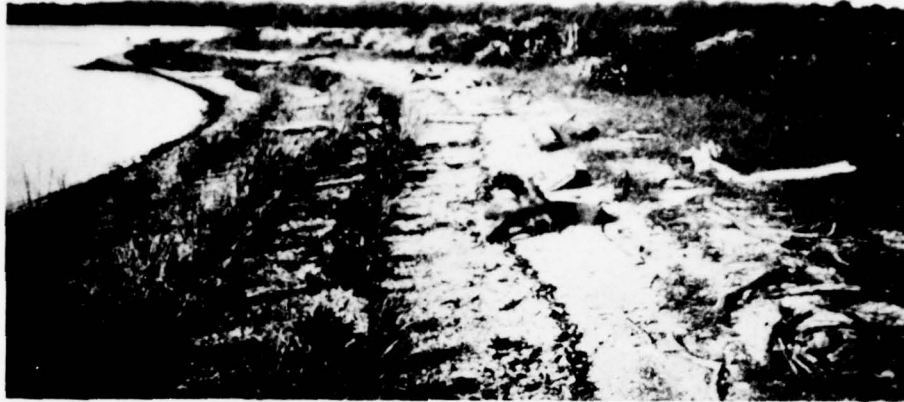
a. EXTERIOR SLOPE, OCT 1975
