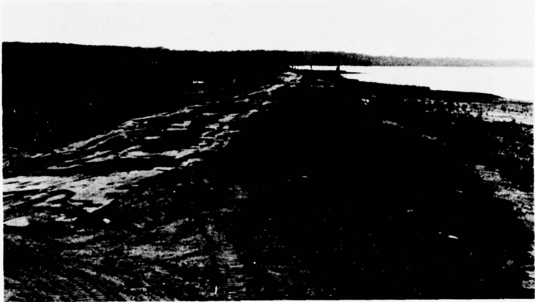
Figure 18. Northeast corner of the dike looking west along the north side on 31 July 1975 just following seeding (after Garbisch 1978).
