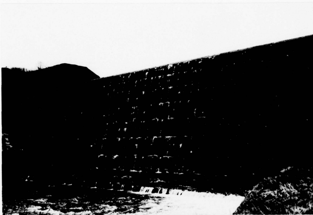
DOWNSTREAM SLOPE OF SPILLWAY SHOWING SEEPAGE FLOW [OBSERVATION (L)] (CARMEL MAIN DAM)
