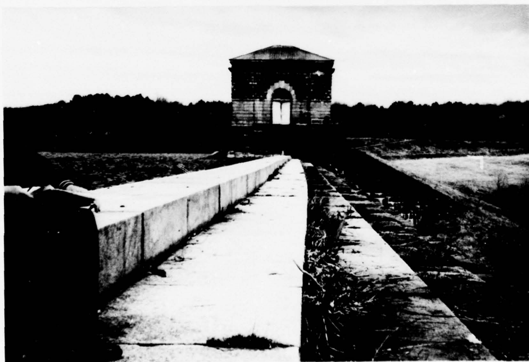
SPILLWAY CREST, DISLOCATED STONES OF THE UPPER TWO COURSES AND SEEPAGE FLOW ARE SHOWN [OBSERVATIONS (M) AND (L)] (CARMEL MAIN DAM)
