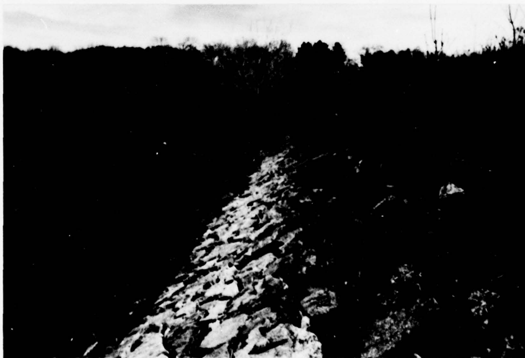
UPSTREAM SLOPE PROTECTION. SOME VEGETATION GROWTH IS SHOWN. [OBSERVATION (A)] (CARMEL MAIN DAM)
