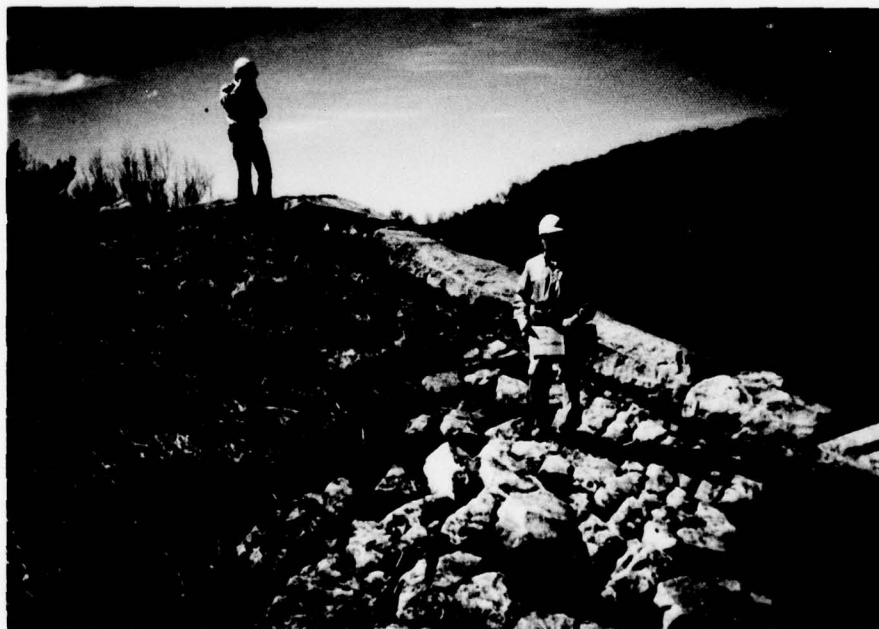
DOWSLOPE MOVEMENT OF RIPRAP, SOUTH EMBANKMENT
