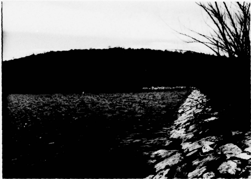
UPSTREAM SLOPE OF NORTH EMBANKMENT
