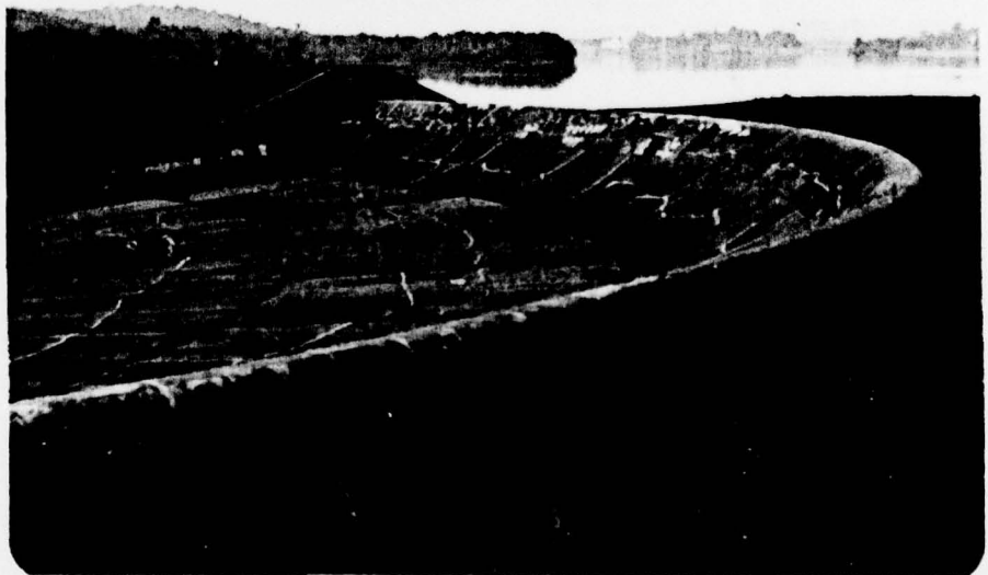
Photograph No. 2 Spillway crest.
