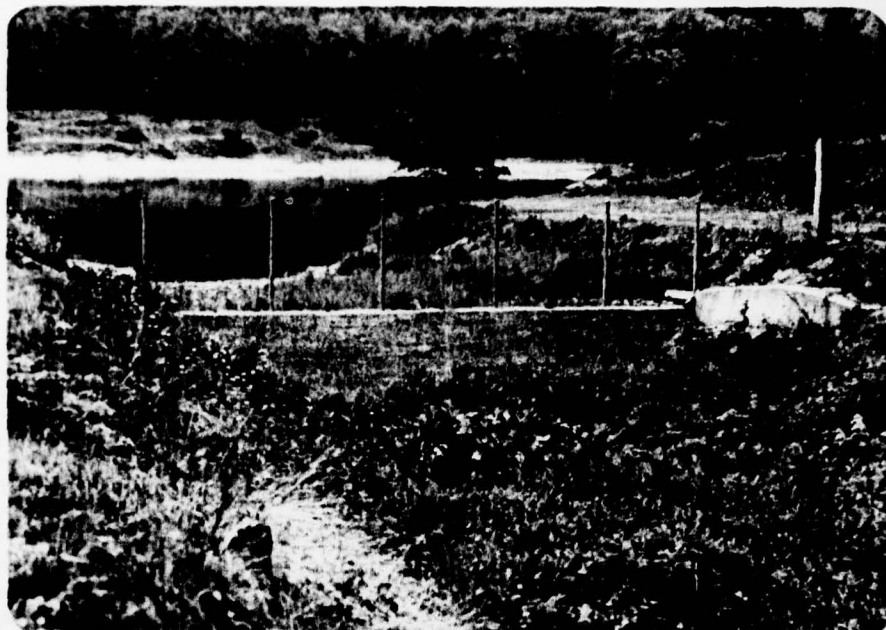
Photograph No. 3 Spillway crest.
