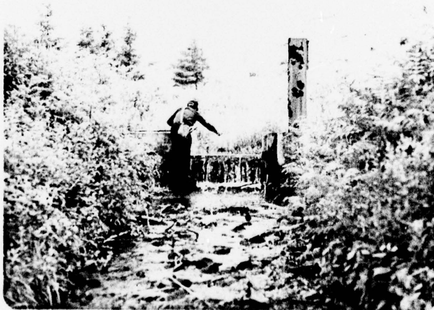
Photograph No. 8 Seepage weir.
