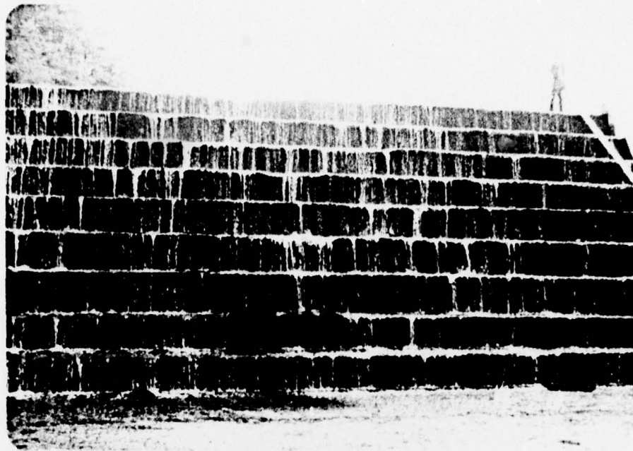
Photograph No. 3 Spillway discharge channel.
