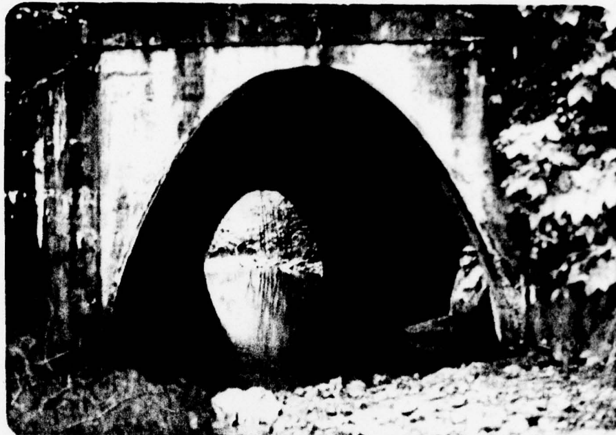
Photograph No. 7 Culvert under Route 422 (looking downstream).
