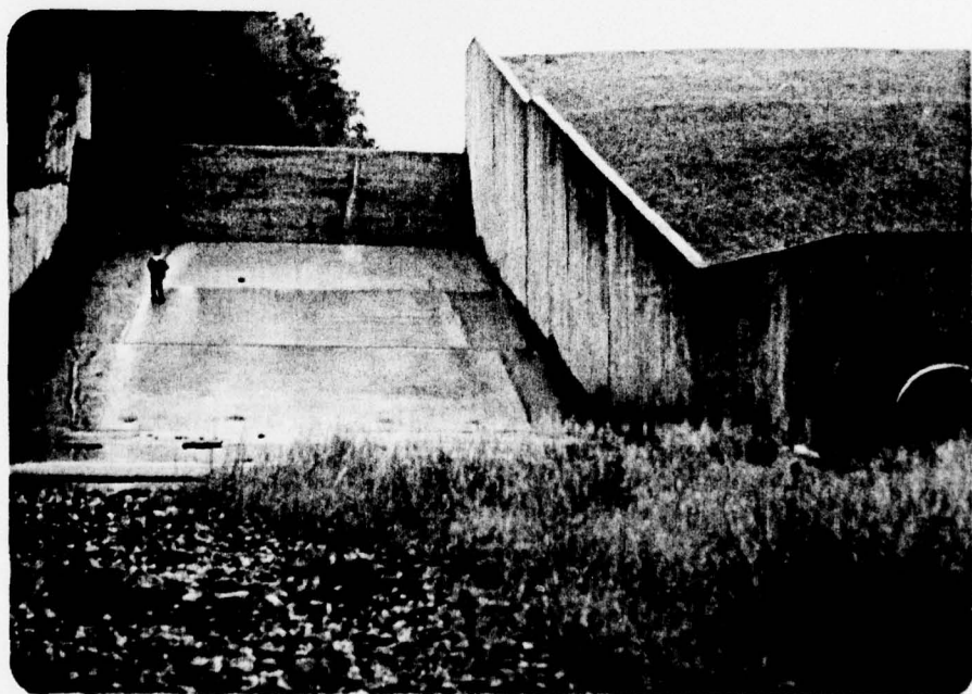
Photograph No. 4 Spillway chute (note drainpipe outlet on righthand side).
