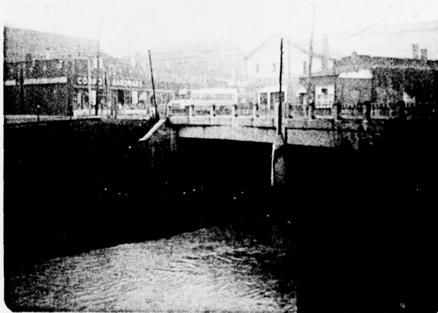
Photograph No. 8 South Branch of Black Lick Creek at Nanty Glo (six miles downstream).
