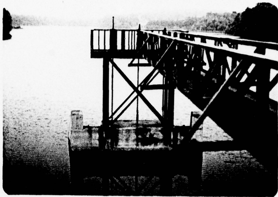
Photograph No. 5 Upstream valve controls.
