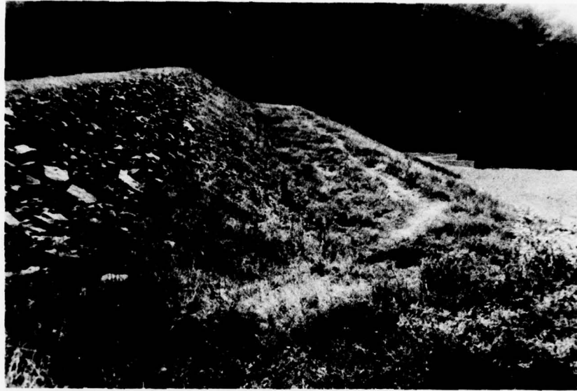
E. Downstream Slopes of Embankment. View from Right Abutment.
