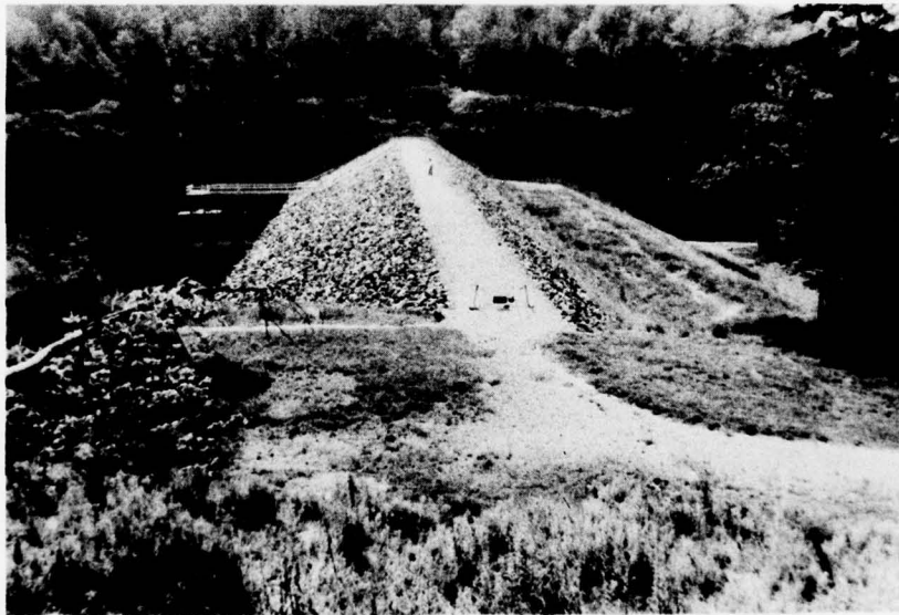
B. Embankment. View from Right Hillside.
