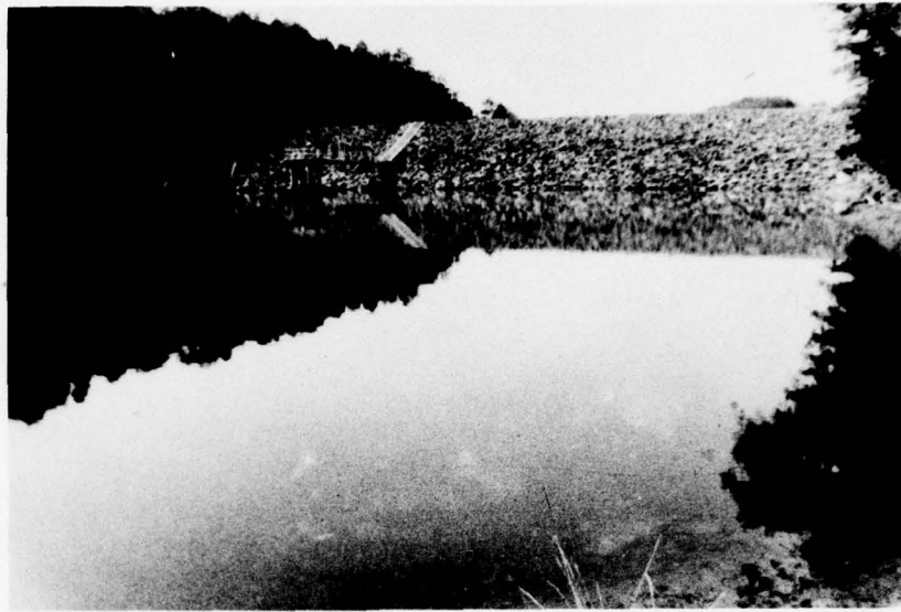
A. Embankment. View from Upstream.
