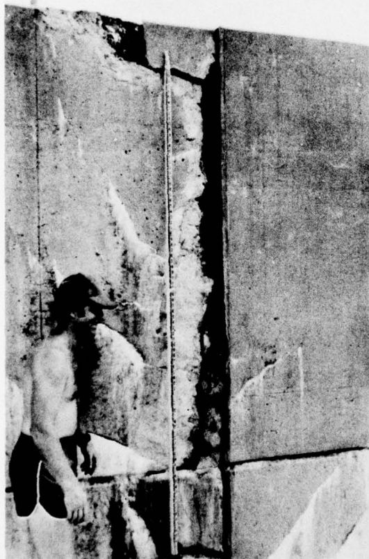
J. Concrete Ogee and Right Training Wall Showing Monolith Cracking and Spalling at Joint.
