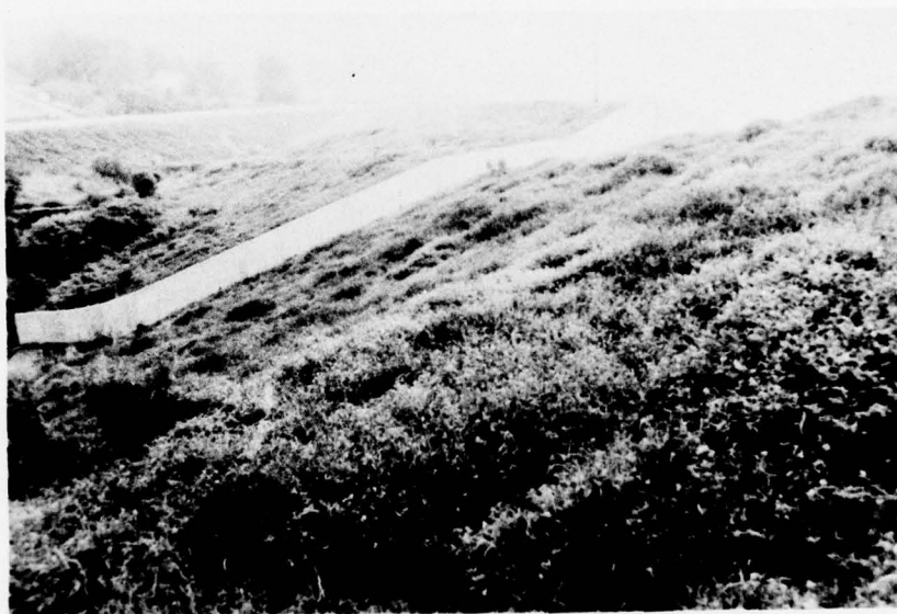
D. Spillway. Embankment in Background.
