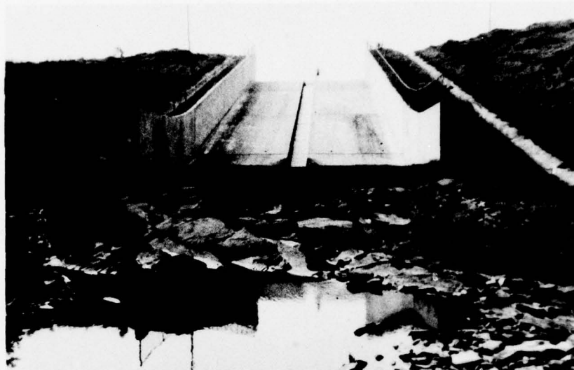
N. Concrete Chute, Flip Bucket, and Paved Gutters.
