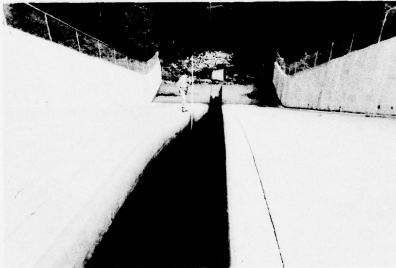
M. Concrete Chute and Flip Bucket.
