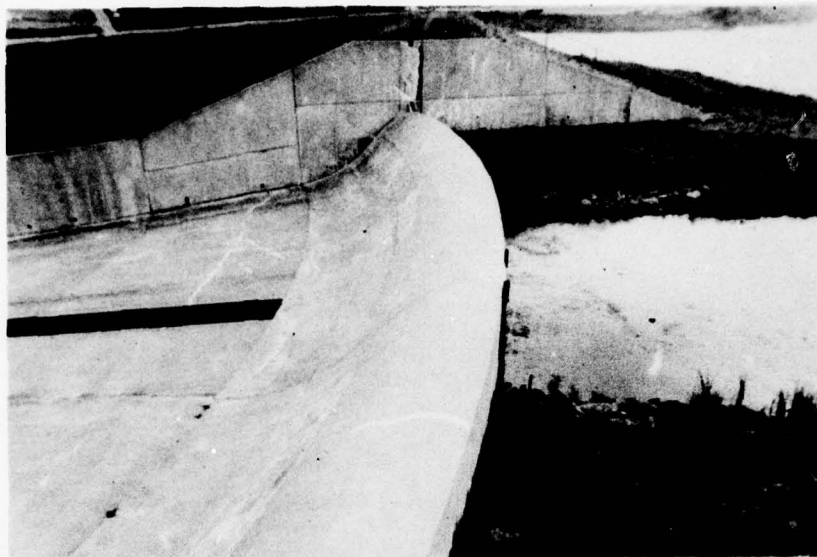
G. Concrete Ogee and Right Training Wall.
