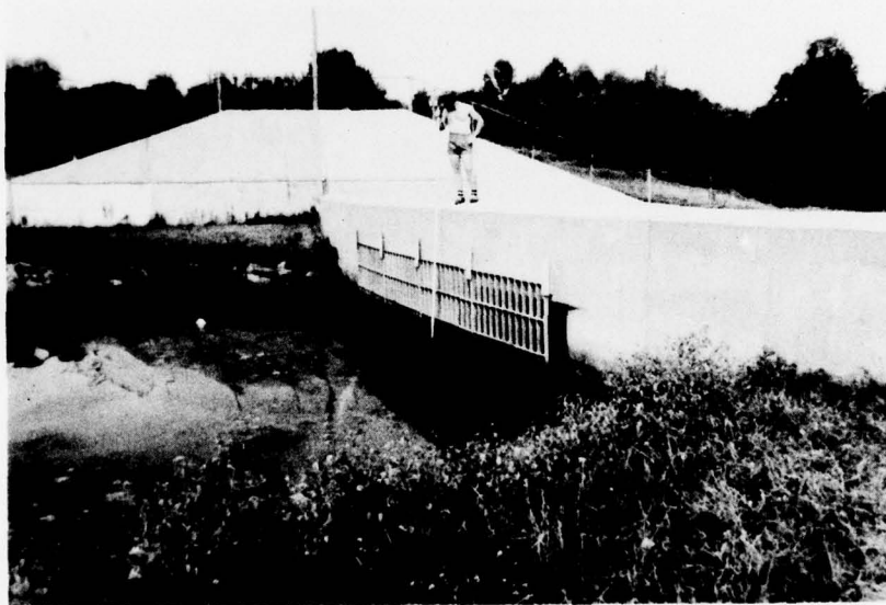
F. Bar Screen Over Low-Flow Opening in Spillway.
