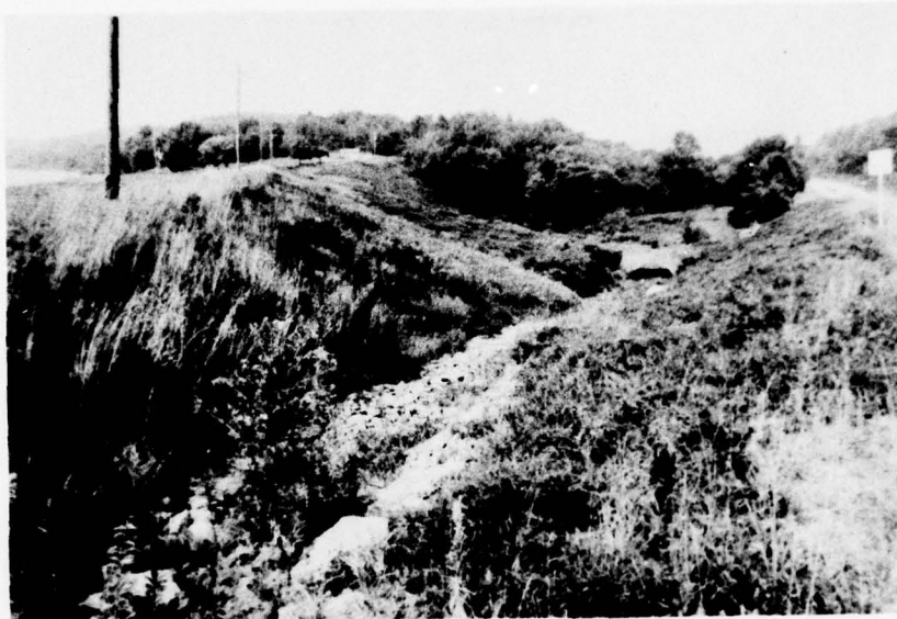
C. Downstream Slope of Embankment. View from Right Abutment.
