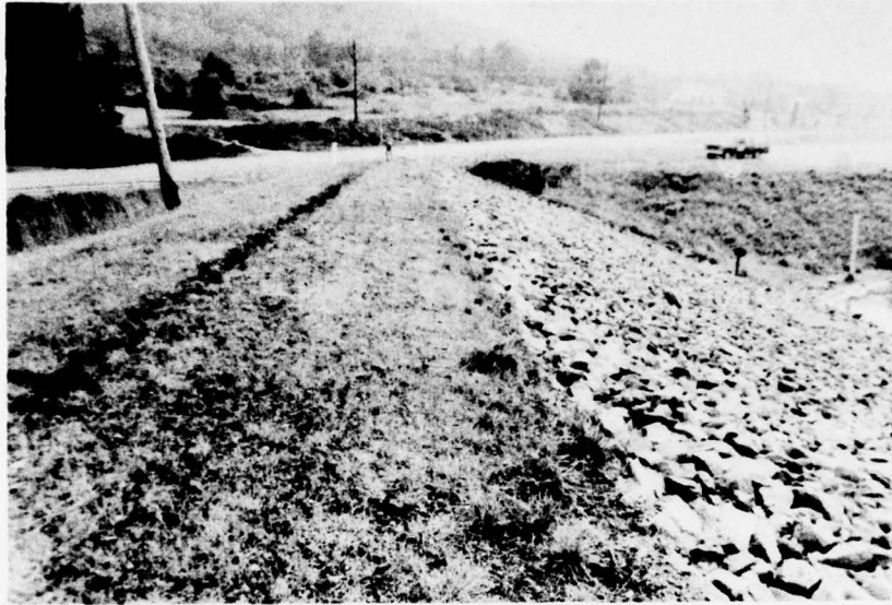
A. Junction of Embankment and Right Abutment. Staff Gages at Right.
