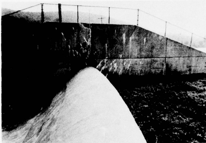
J. Concrete Ogee and Right Training Wall Showing Monolith Cracking and Spalling at Joint.
