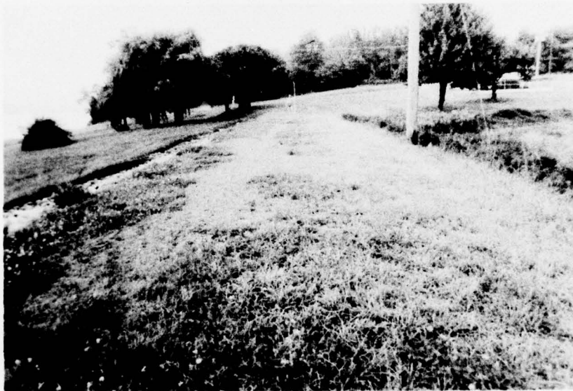
B. Junction of Embankment and Left Abutment.
