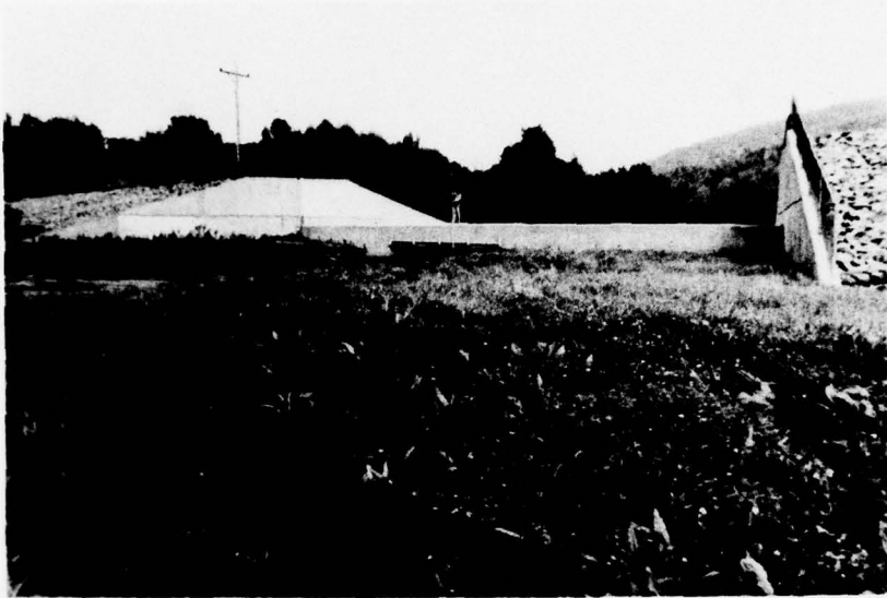
E. Spillway Approach Channel.
