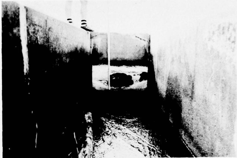
L. Low-Flow Outlet at Downstream Side of Spillway Weir.
