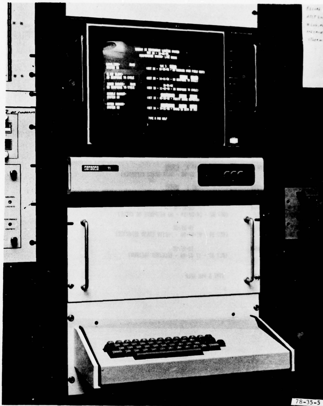
FIGURE 5. CENTRAL MICROCOMPUTER AND DISPLAY UNITS AT THE CONTROL TOWER
