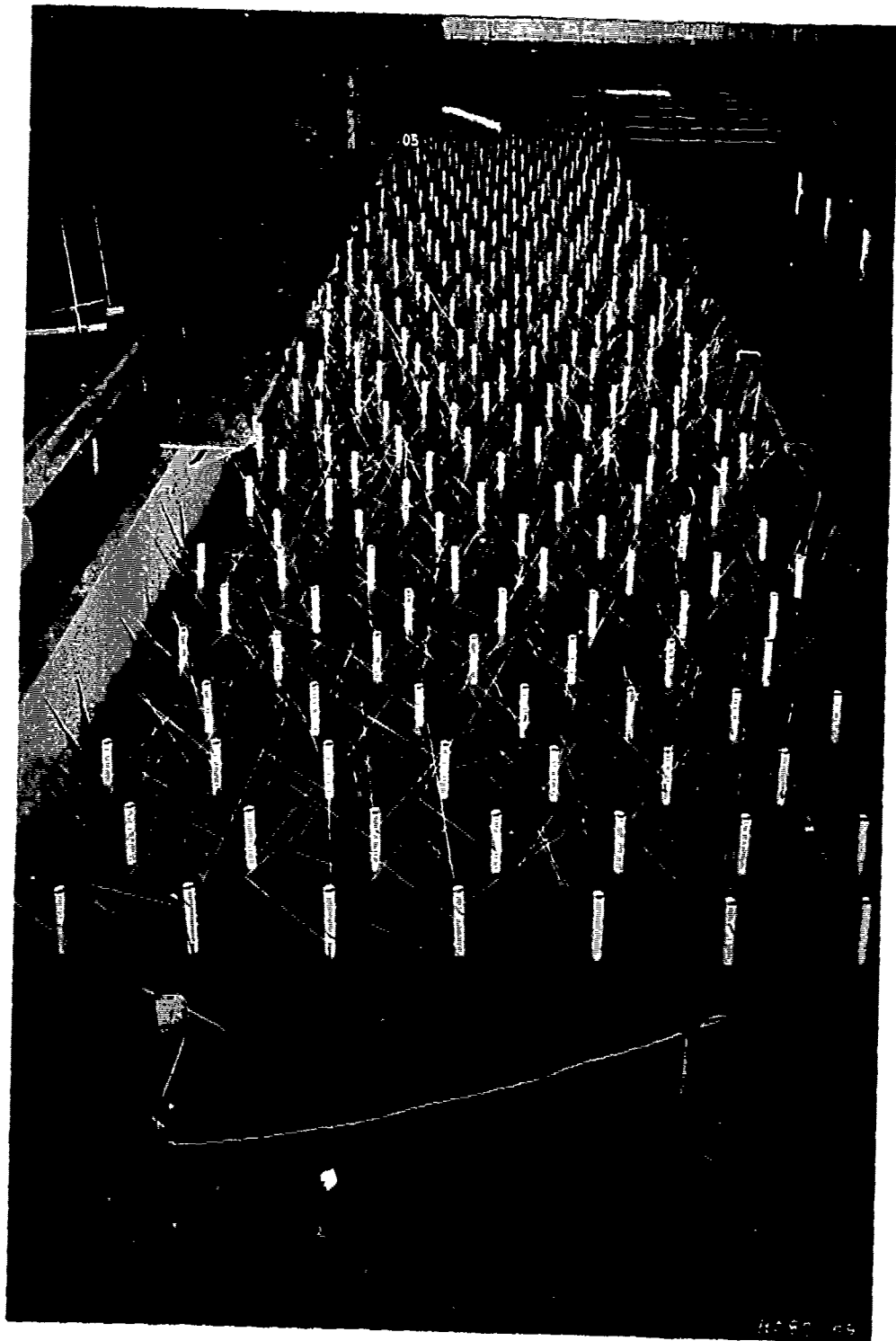
Photo 8. Plan 12, 12-in.-diameter stems with 1-1/4-in. branches with model water depth of 2.0 ft
