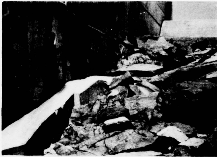
Spillway Chute Wall Toe Protection
