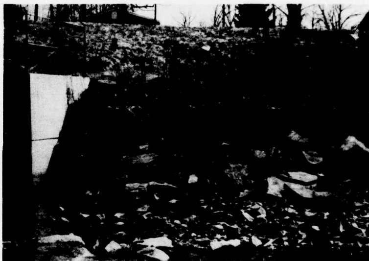
Left Wall Stilling Basin
