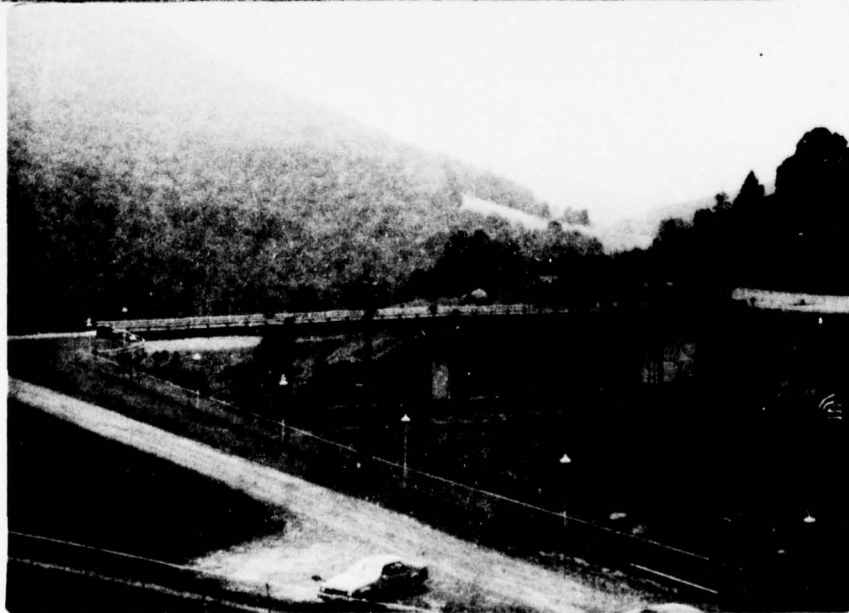
Forebay and Spillway Bridge
