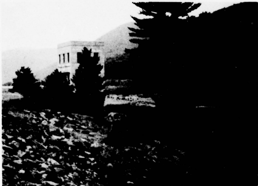
Reservoir and Tower
