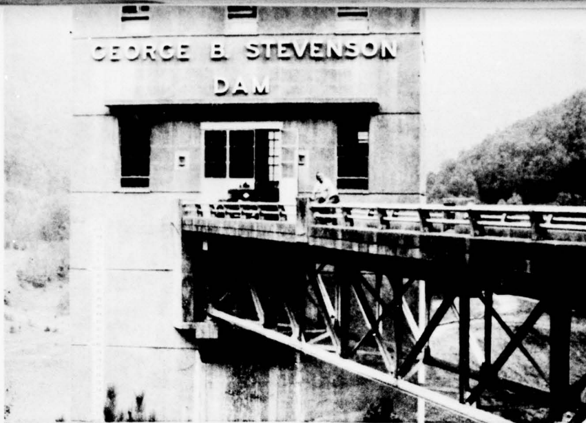
Access Bridge to Tower
