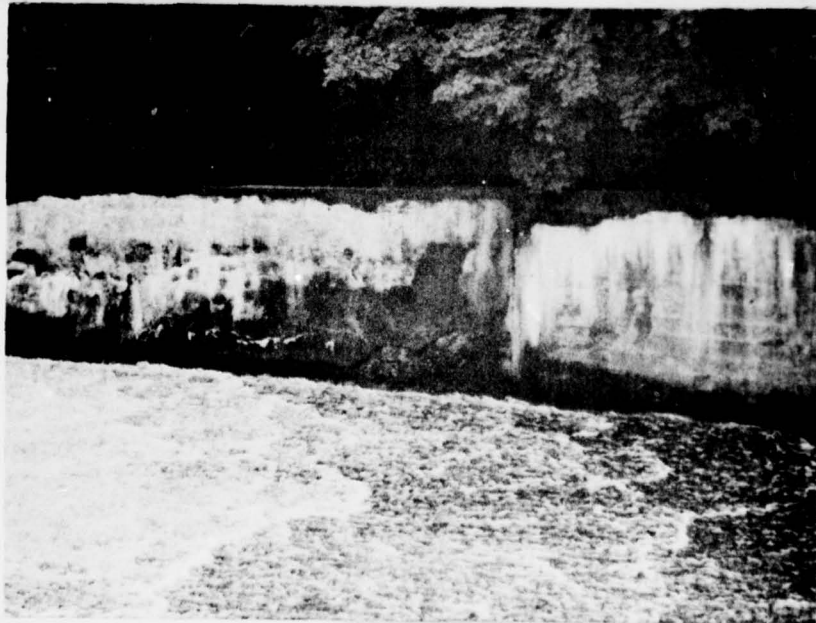
Walls of Spillway
