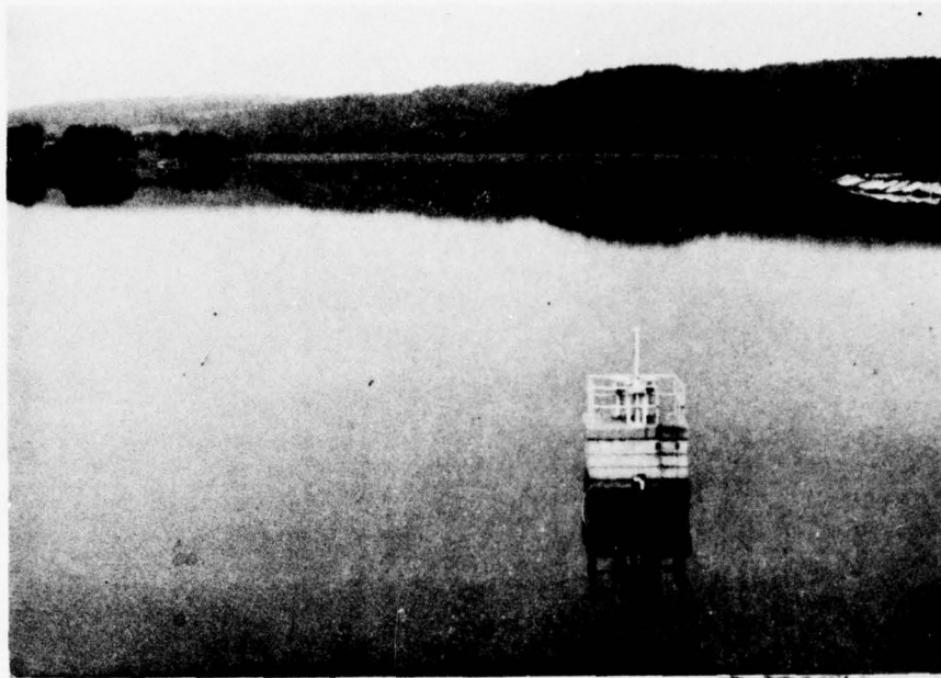
Reservoir and Intake Tower
