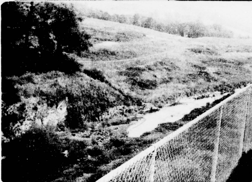
Spillway Channel Looking Downstream
