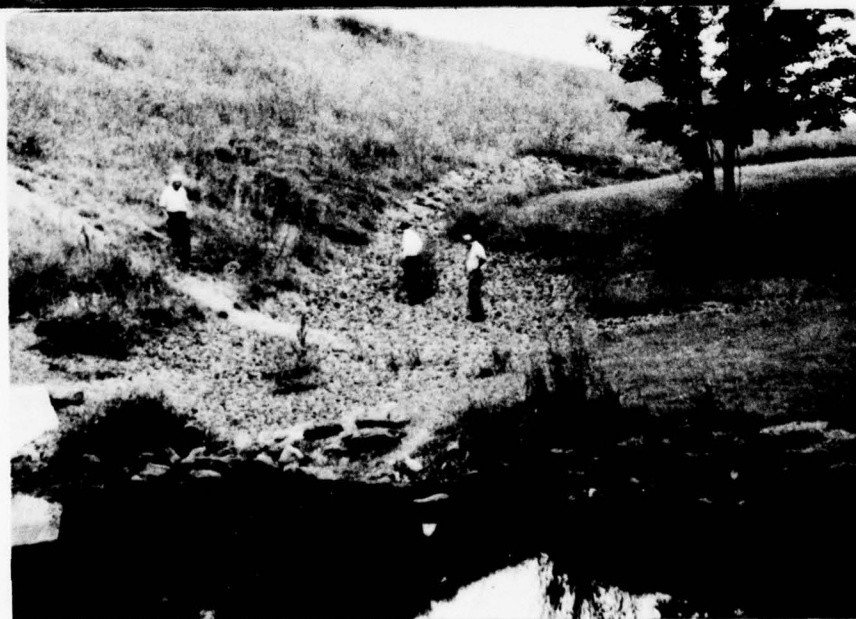
Toe Near Conduit Outlet
