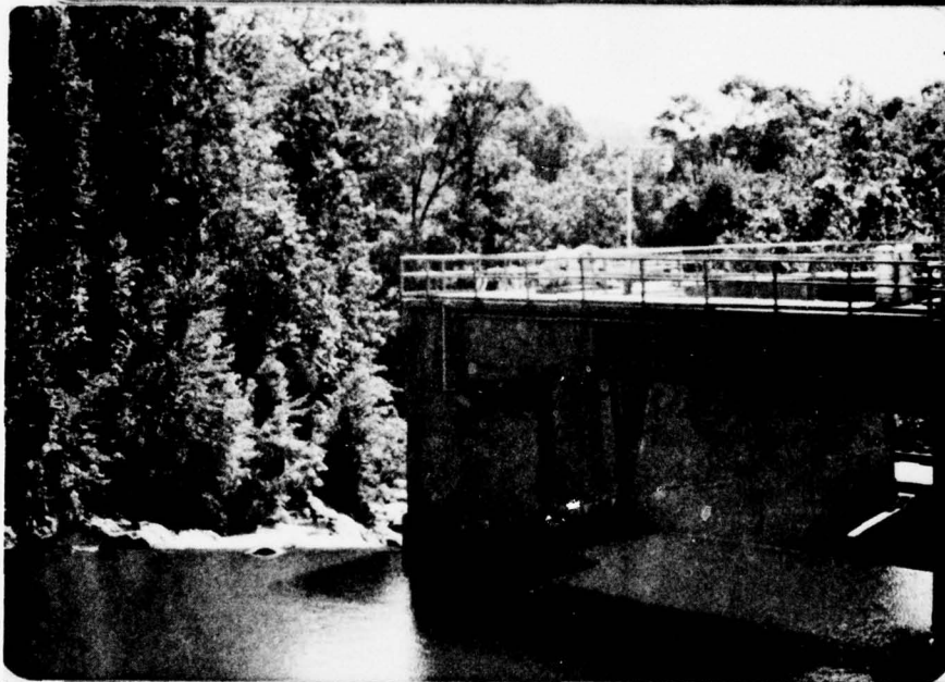
Spillway and Tainter Gate
