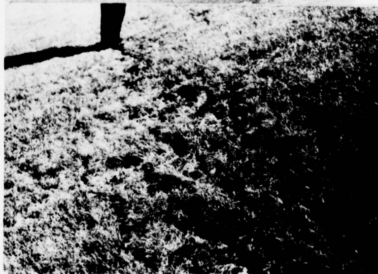
Embankment Slope "Mole Activity"
