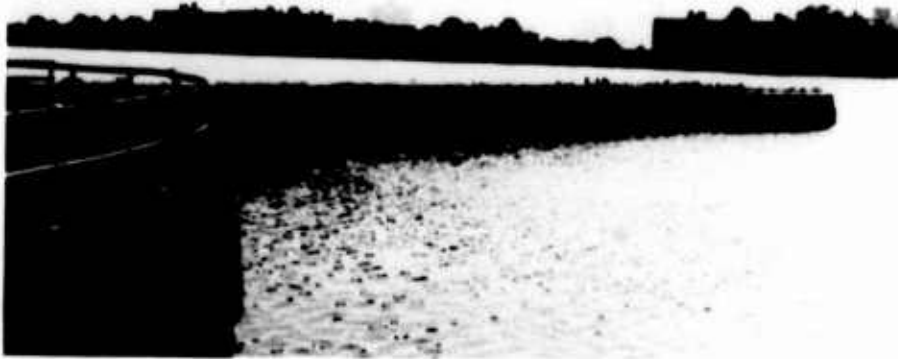
FIGURE 9 VIADUCT LEADING FROM GATEHOUSE No. 5 (LEFT) TO SHAFT No. 21 (RIGHT)
