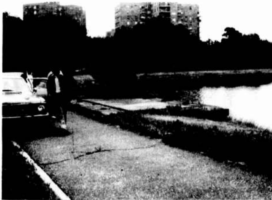
FIGURE 5 WASTE WIER AND SECTION OF RETAINING WALL AND EMBANKMENT ON WESTERN SIDE OF RESERVOIR
