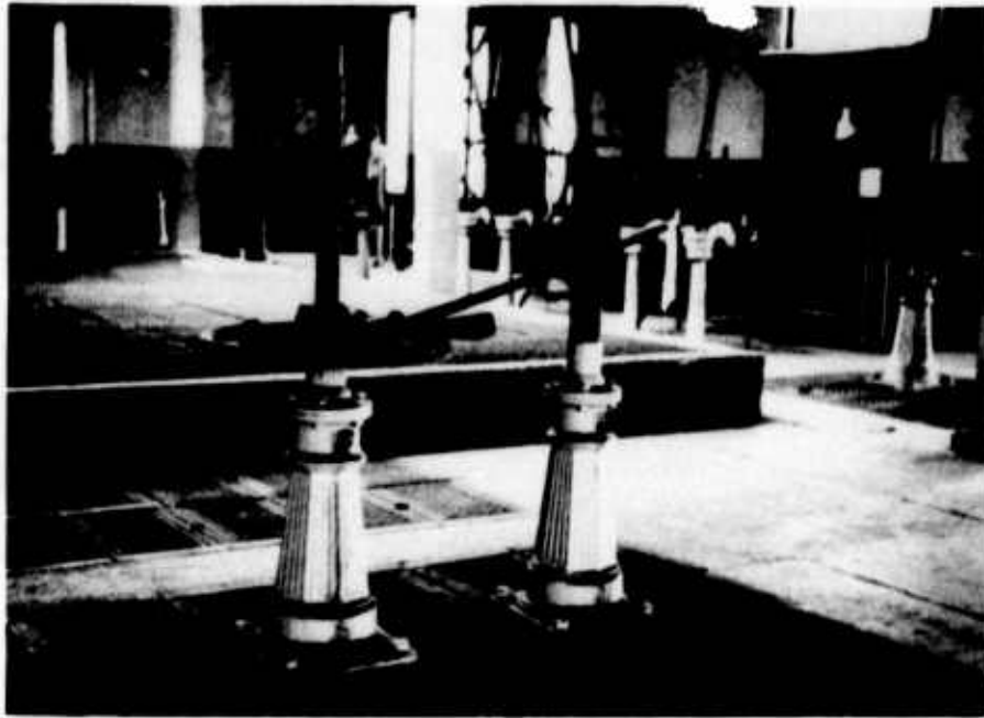
FIGURE 7 GATEHOUSE No. 5 GATE STAND ARRAYS
