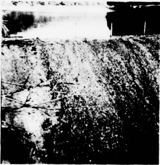
4. Closeup of spillway surface which is in serviceable condition with some surface erosion.
