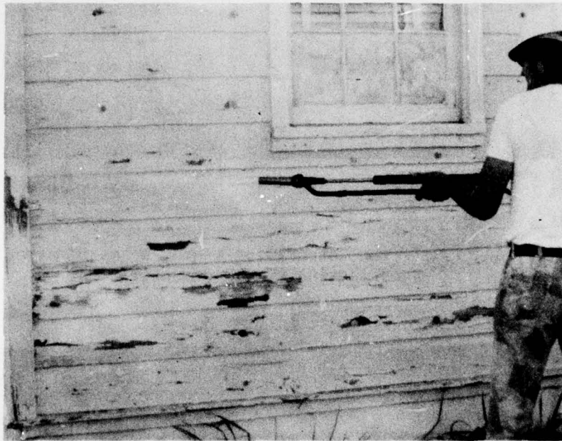
Figure 3. Hydroblaster being used to clean World War II mobilization building.
