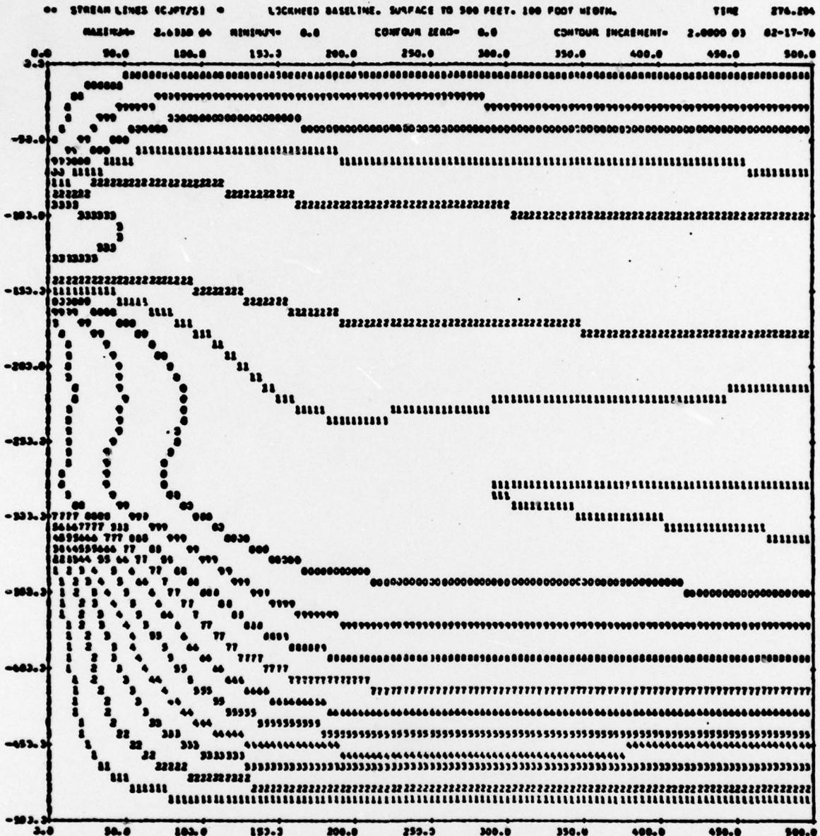
**Figure 4.** Streamlines for steady 2-D flow designed to simulate a Lockheed baseline plant. The portion of the computational domain shown is a vertical cross-section 500 ft in depth and 500 ft in horizontal extent. The intake is at 50 ft depth and the warm and cold discharge are located at 150 and 300 ft. The inflow and outflow ports each occupy 75 ft in the vertical. The density profile is typical of the Gulf of Mexico in August.
