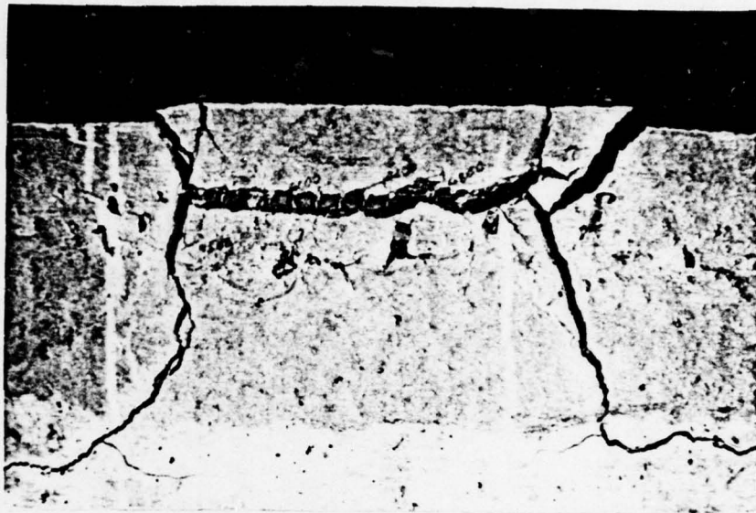
Fig. 27. This is the final position of the crack formation for Beam T-2-P. The block of PCC which was lifted from the splice zone was not loose and could not be picked up from the beam.
