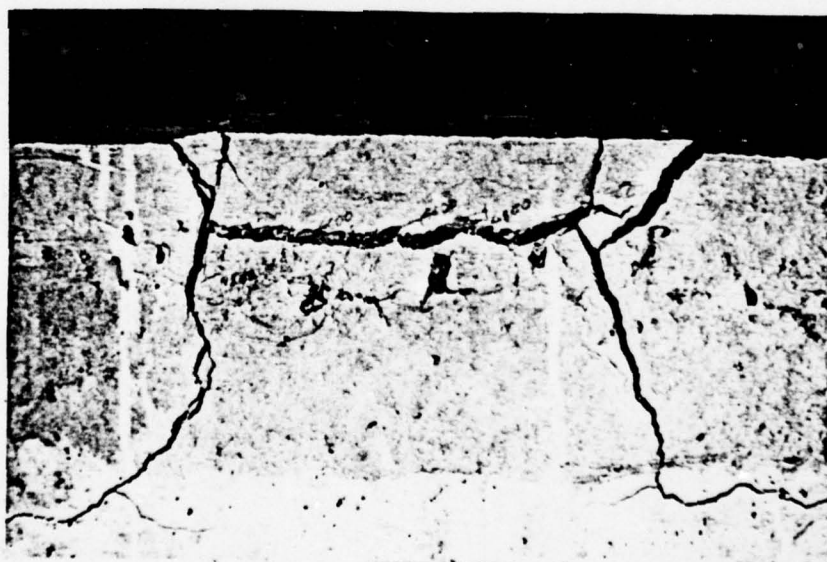
Fig. 26. The beam continues to deform with the PCC material in the splice zone visibly lifting from the beam. Note the extension of the vertical cracking from the splice zone to the compression steel.
