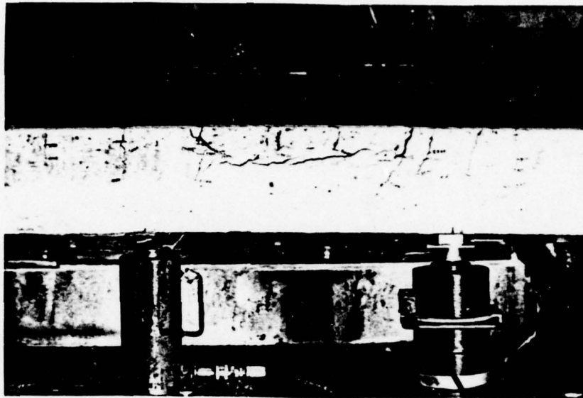
Fig. 17. Failure of T-3-C. Splice length = 16 inches. Ultimate load = 6.5 kpj. Note the supplementary flexure cracks near the third points of the splice length.
