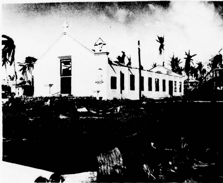
Figure 16 - Structural damage suffered by Talofofo church due to Karen's winds (photo by V. Olsen)
