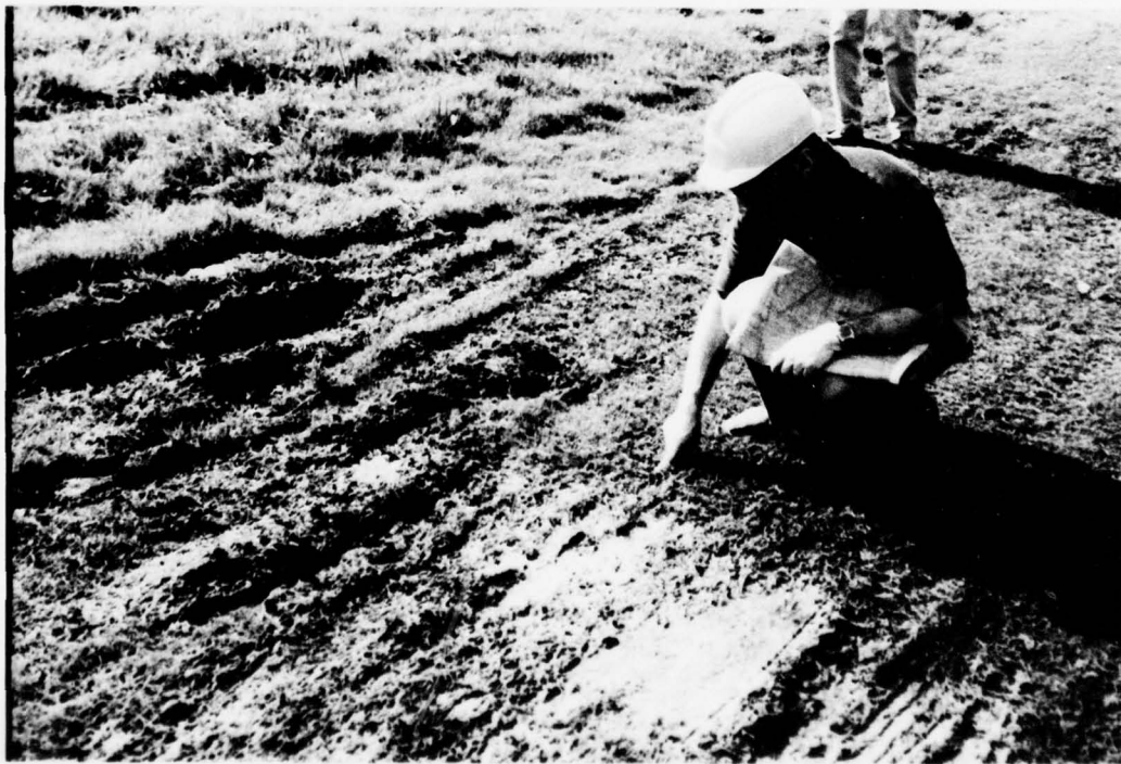
WET AREA AT BERM LEVEL (EL 218 + ) OF NORTH DIKE
