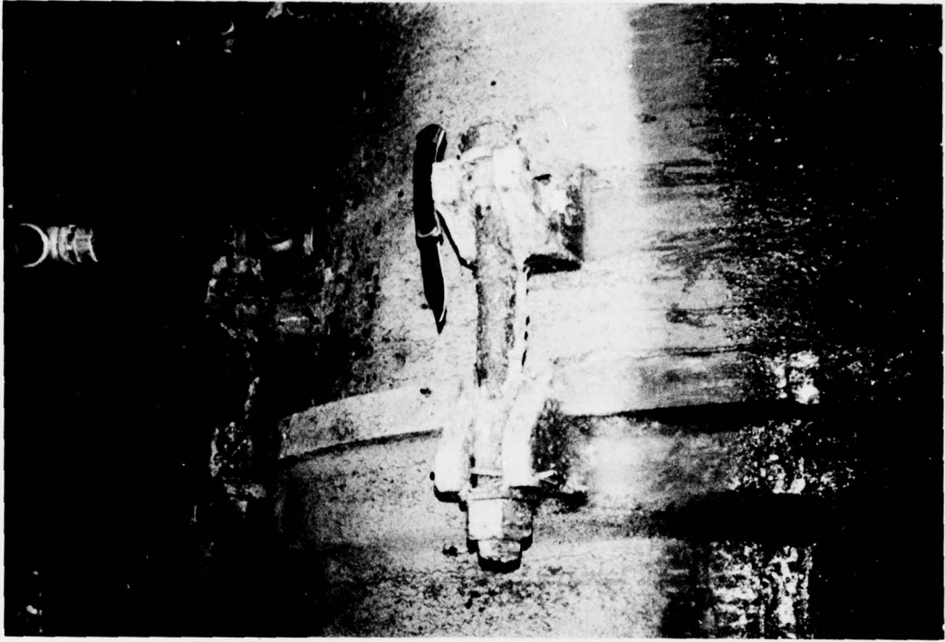
CORRODED TIE RODS (TYPICAL) CON- NECTING CONDUIT TO 48 INCH CAST IRON MANIFOLD
