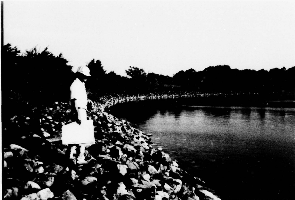
UPSTREAM SLOPE OF NORTH DIKE, LOOKING NORTH
