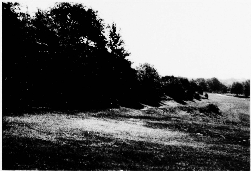
DOWNSTREAM SLOPE OF SOUTH DIKE, LOOKING EAST. CREST IS NOT VISIBLE; FLAT AREA IS BERM AT EL 218±
