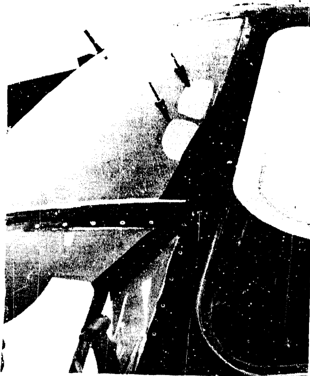
Figure 110. CH-53, External View of Delaminations.
