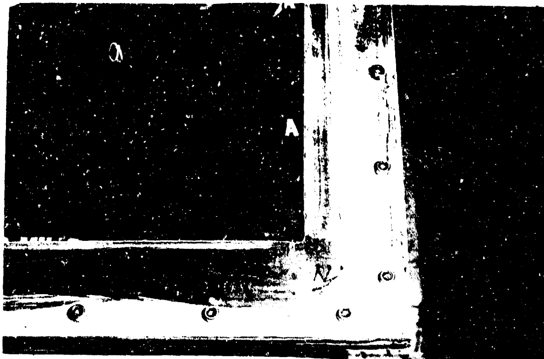
Figure 168. Bolted Attaching Arrangement.
