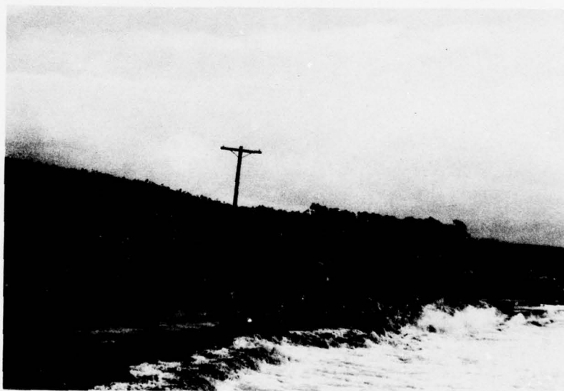
FIGURE 24 - BLUFF EROSION THREATENING COASTAL HIGHWAY 1 NEAR HALF MOON BAY, CA
