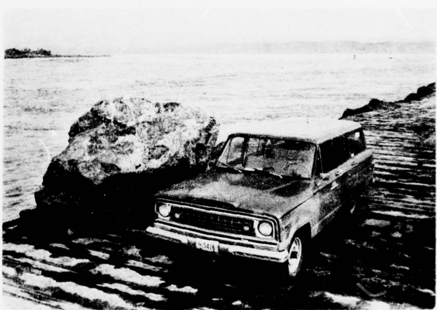
FIGURE 18 - DISPLACED 20 TON BOULDER, HUMBOLDT HARBOR JETTY
