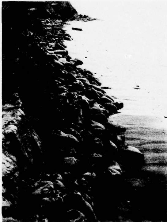
FIGURE 22 - SANDBAGS PROTECTING THE DUNE SCARP AT SEADRIFT SPIT
