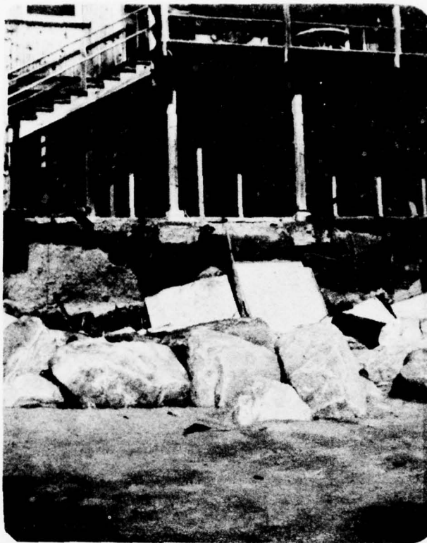
FIGURE 25 - ERODED FOUNDATIONS AT POTBELLY BEACH, CA
