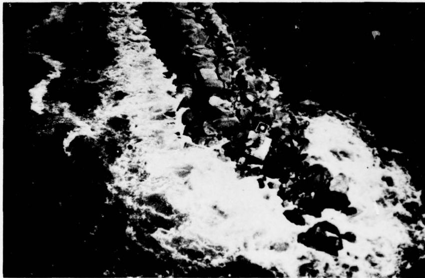
FIGURE 32 - SOUTH JETTY, OCEANSIDE HARBOR
