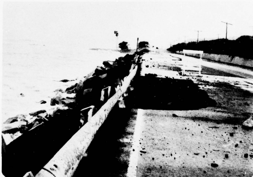
FIGURE 36 - WAVE DAMAGE, OLD COAST HIGHWAY VENTURA COUNTY, CALIFORNIA
