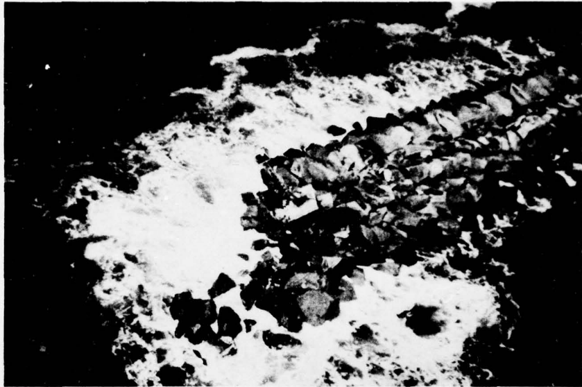
FIGURE 31 - SOUTH JETTY, OCEANSIDE HARBOR
