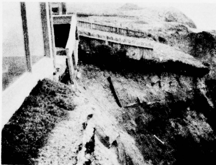
FIGURE 23 - CLIFF EROSION AT PACIFICA, CA
