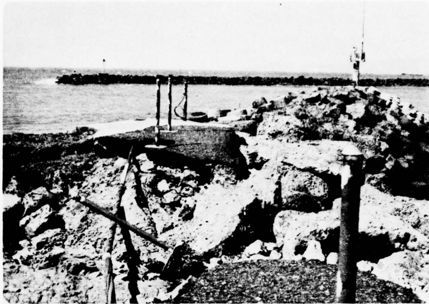
FIGURE 35 - DAMAGE TO WALKWAY AT VENTURA MARINA
