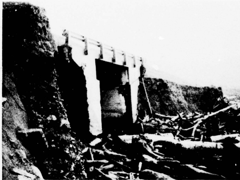
FIGURE 19 - MORGAN POINT BRIDGE NEAR CAPE MENDOCINO, CALIFORNIA
